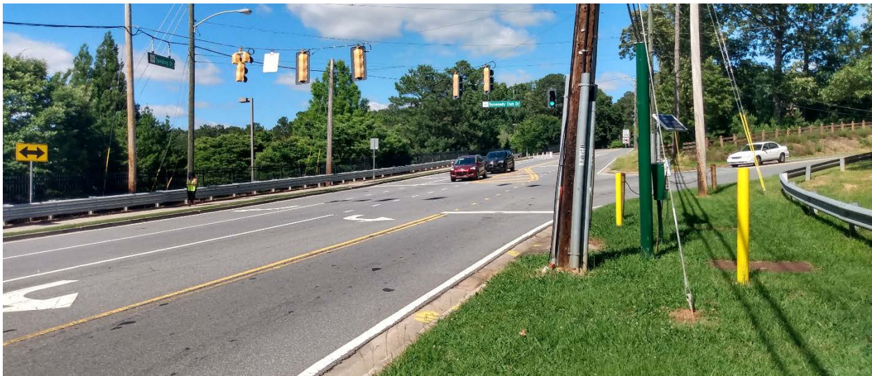
Figure 17: View of Skewed Intersection of Spalding Drive with Dunwoody Club Drive
