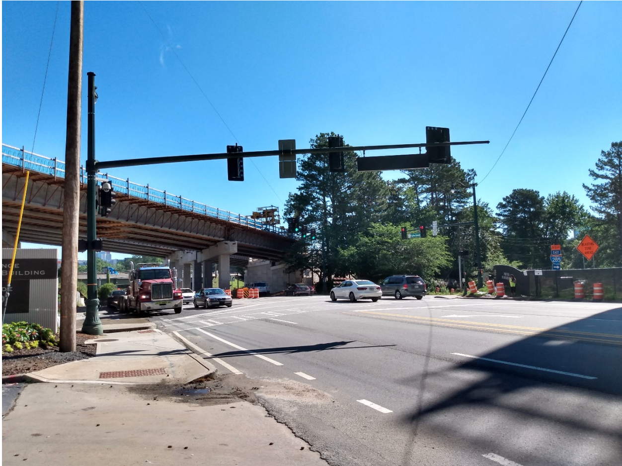
Figure 20: View of Peachtree Dunwoody Rd at Lake Hearn Dr with Construction Along I-285 Overhead
