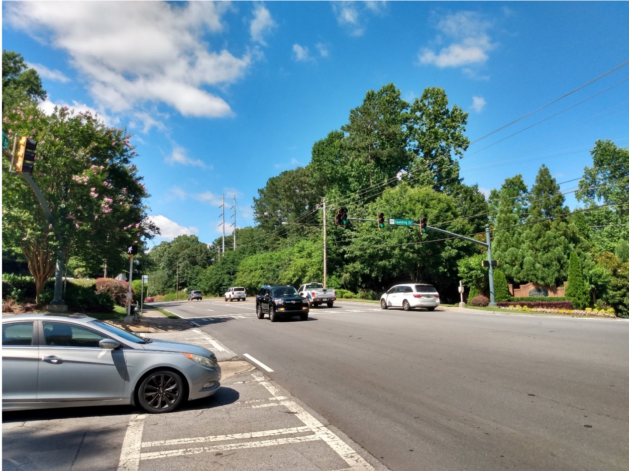
Figure 15: Looking North along Roswell Rd from Spalding Dr
