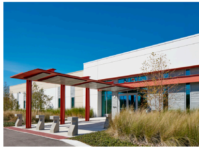
PUBLIC SAFETY OPERATIONS COMPLEX & EMERGENCY OPS CENTER TAMPA, FL
