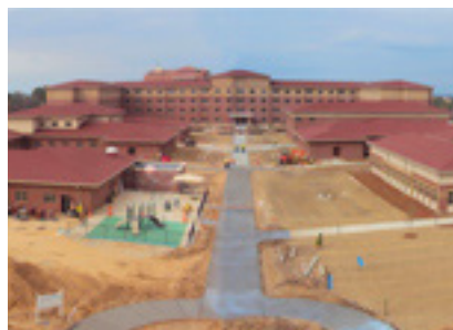
WT ADMINISTRATIVE FACILITIES FORT BRAGG, NC
