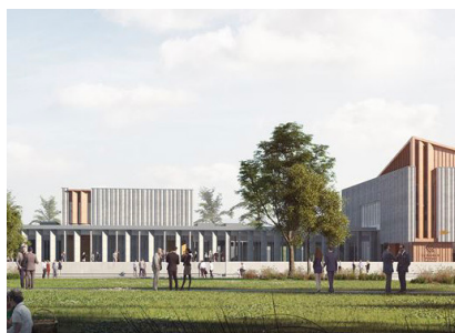
MUNICIPAL CAMPUS SPRINGDALE, AR
