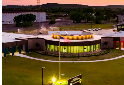
BILLIE A. HALL PUBLIC SAFETY COMPLEX SAND SPRINGS, OK
