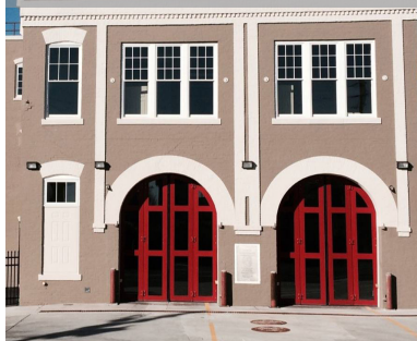
CITY OF ATLANTA Fire Station No. 7
