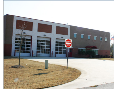
ROCKDALE COUNTY Fire Station No. 1
