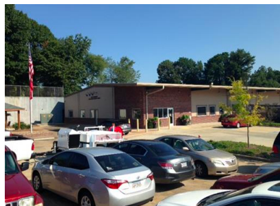
FIRE STATION NO. 2 JEFFERSON, GA
