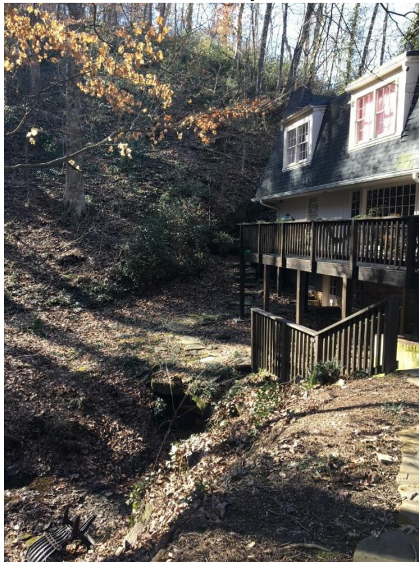
View of culvert and backyard
