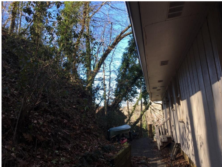
View of cliff in side yard
