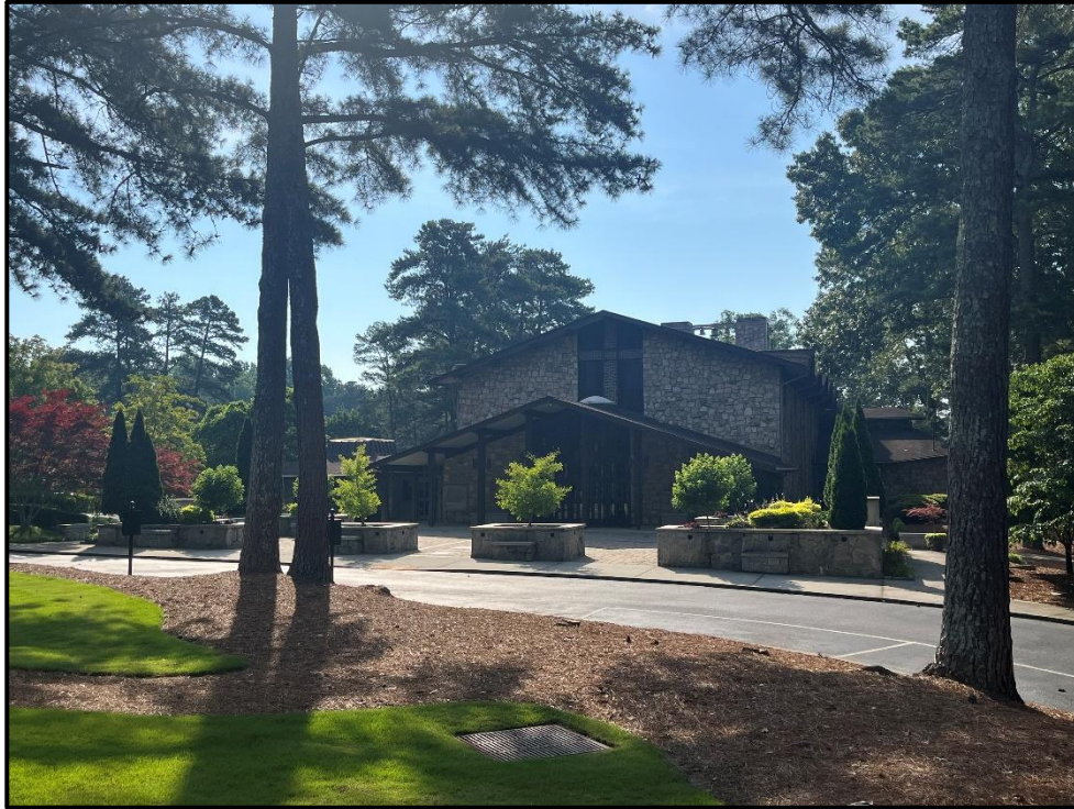
View of the existing Church facing east from Glenridge Drive
