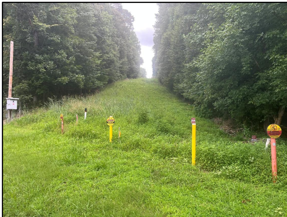
View of pipeline easement on property east of Tanglewood Trail
