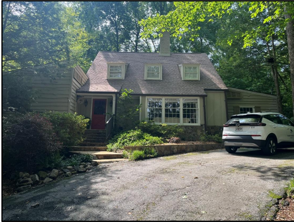
View of the front of the home facing east from driveway
