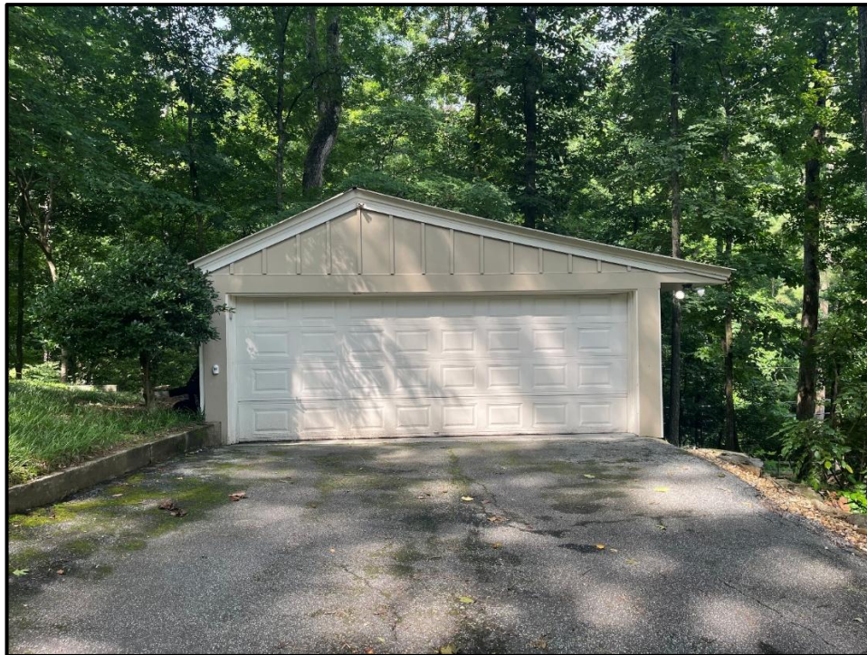
View of the existing garage
