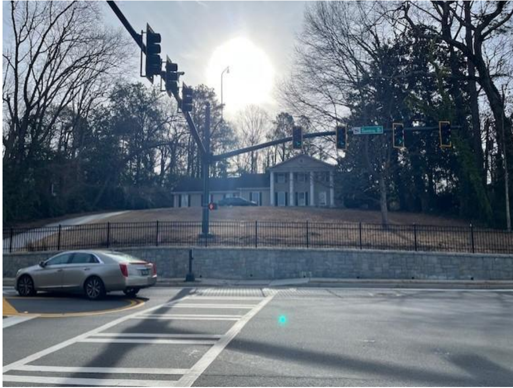
View of 1265 Spalding Drive from Spalding Drive at the Spalding/Pitts signalized intersection
