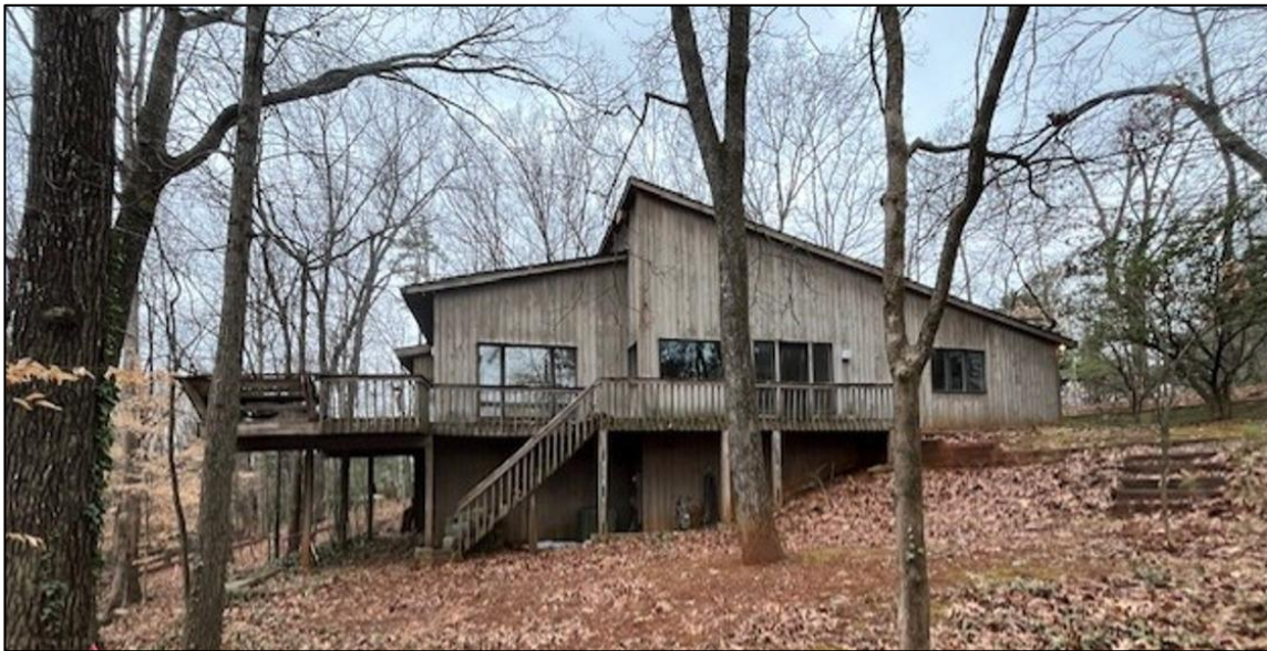
View of home facing west from side yard
