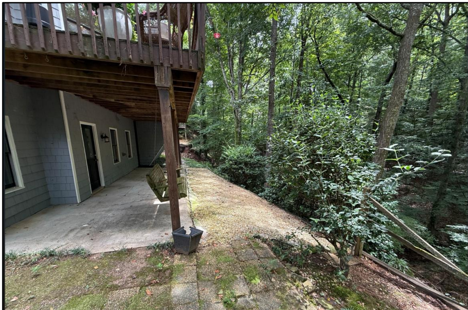
View of rear yard facing southeast*
