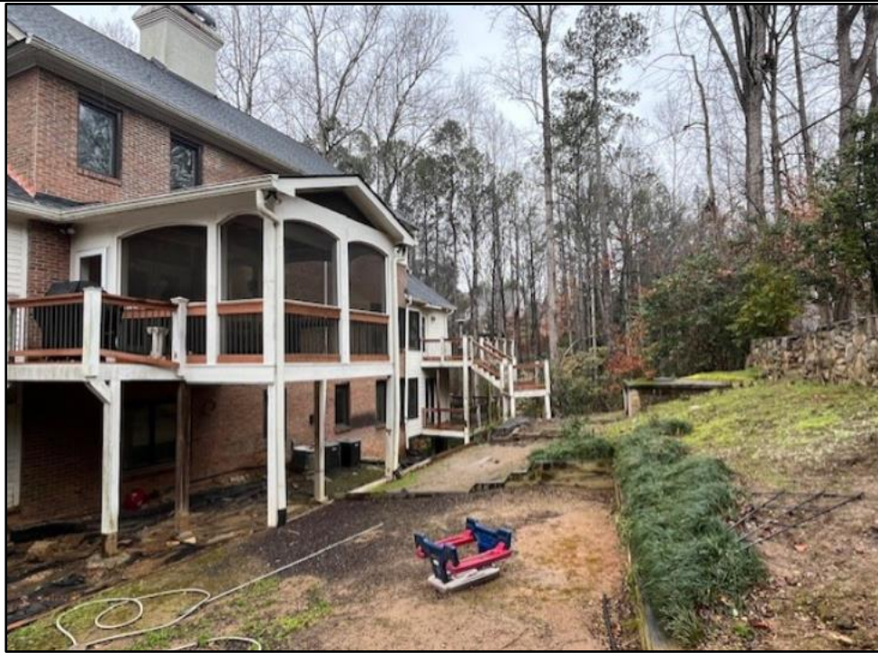
View of rear screened porch and deck to be demolished
