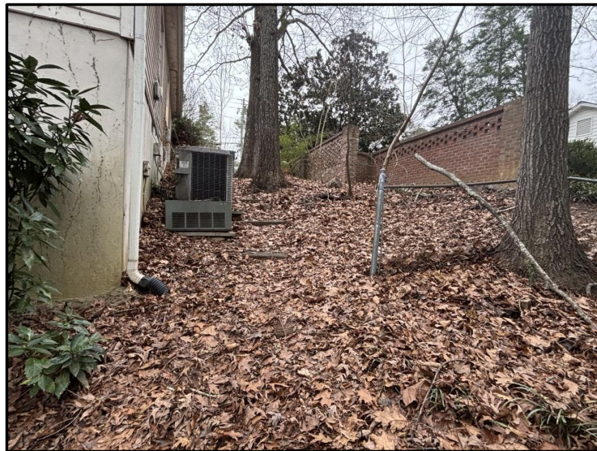
View of west side of home facing South
