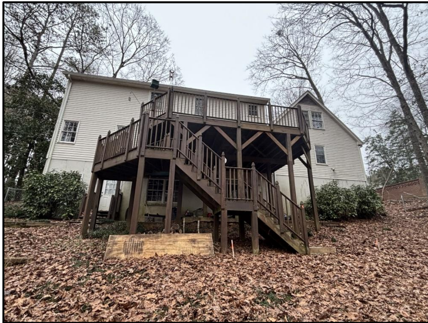
View of rear of home facing South
