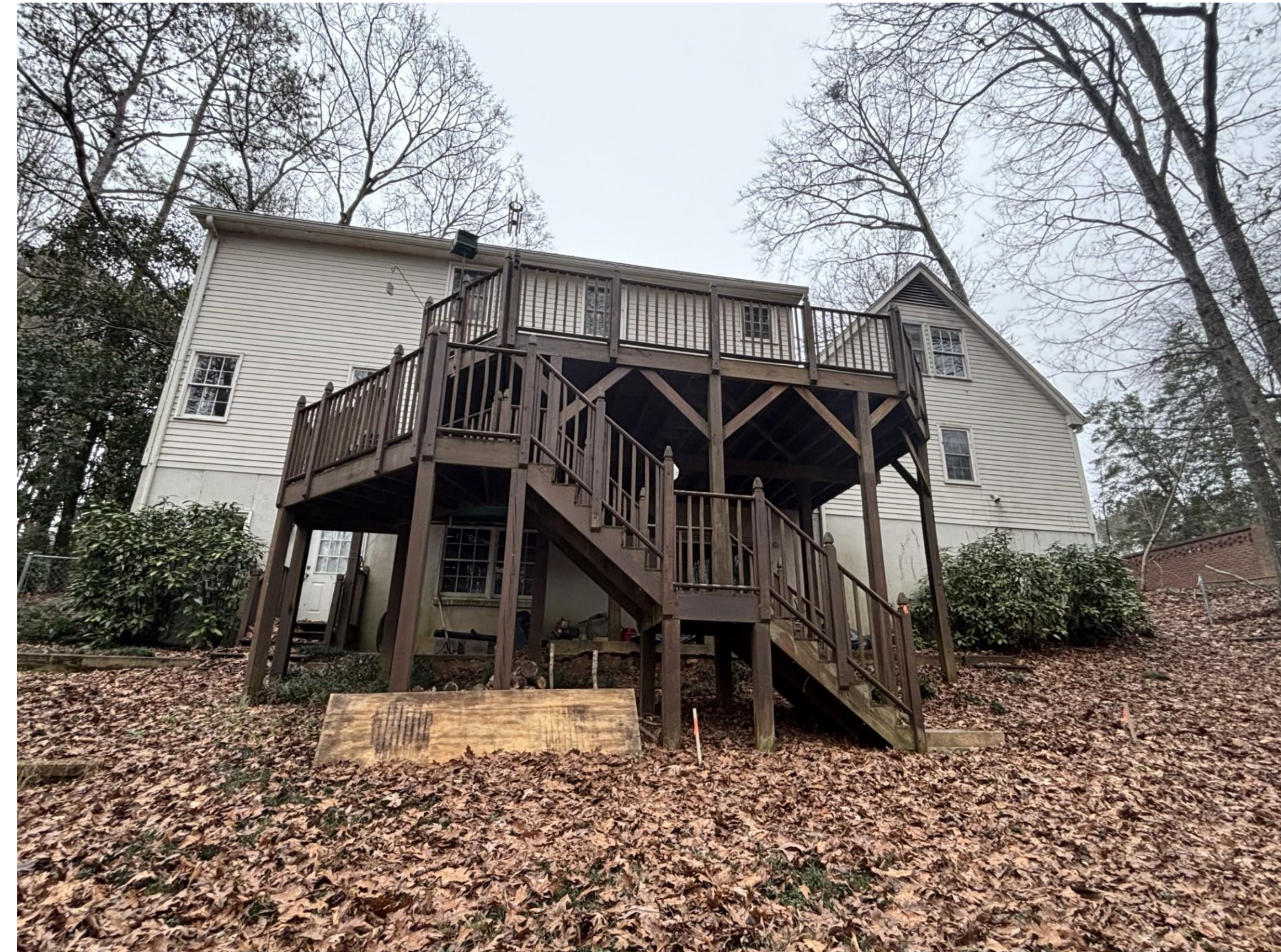
View of rear of home facing south
