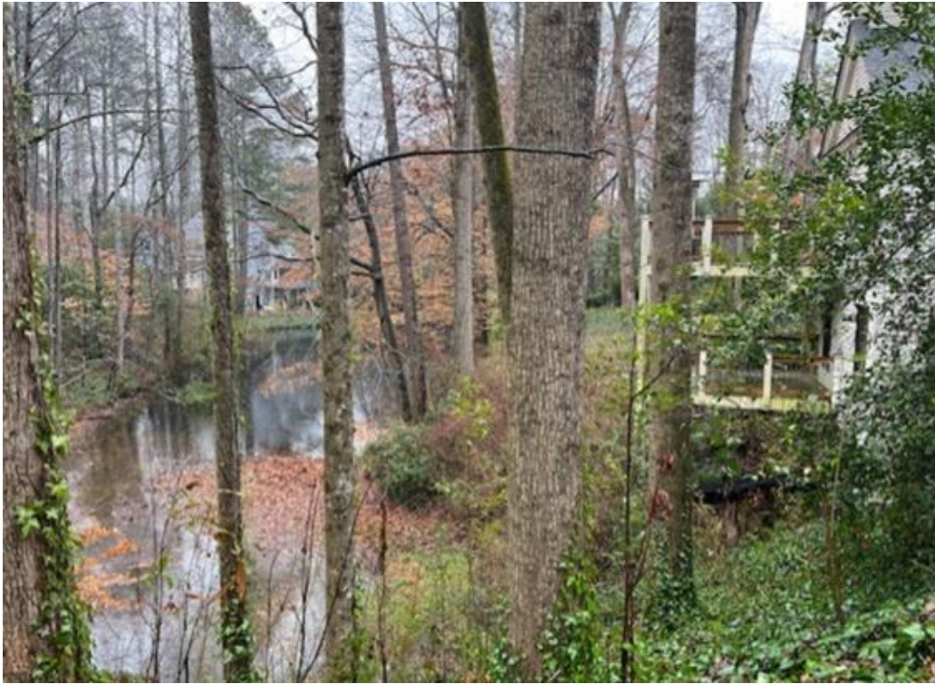
View of slope and partial rear deck standing on Franklin Road facing northeast
