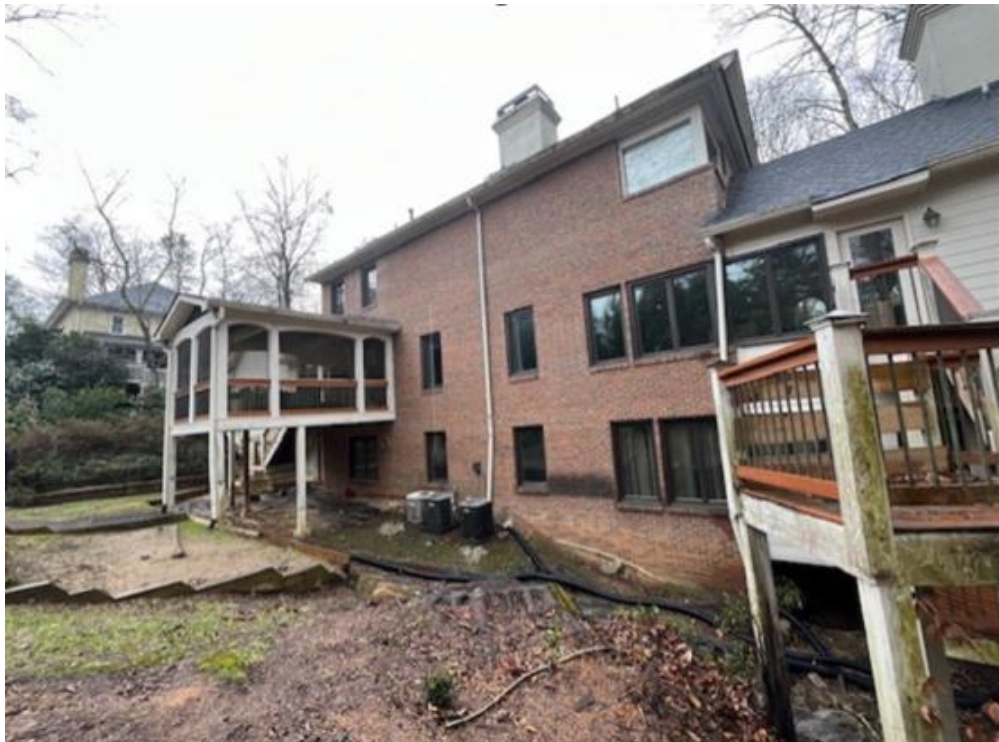
View of existing rear porch
