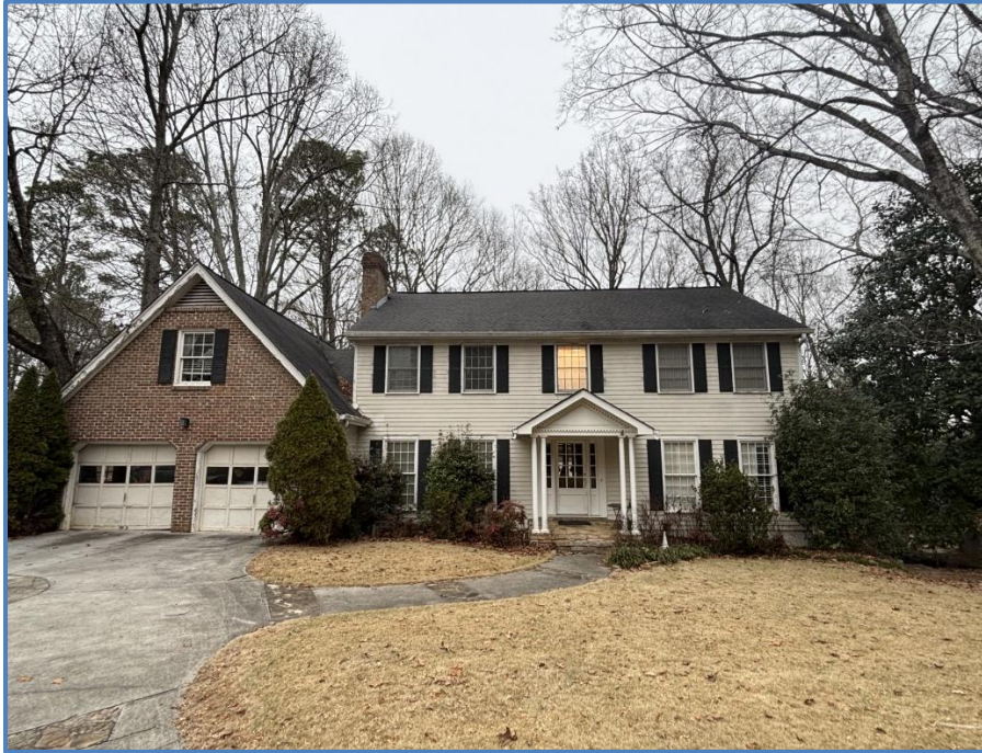
View showing front of home facing North from Edgewater Drive
