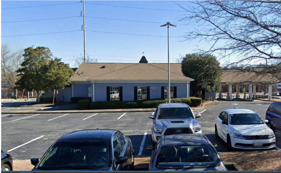
View of rear of existing bank facing east from rear parking lot
