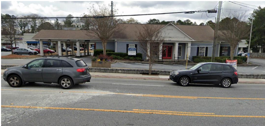
View of the front of the existing building standing on Roswell Road looking west
