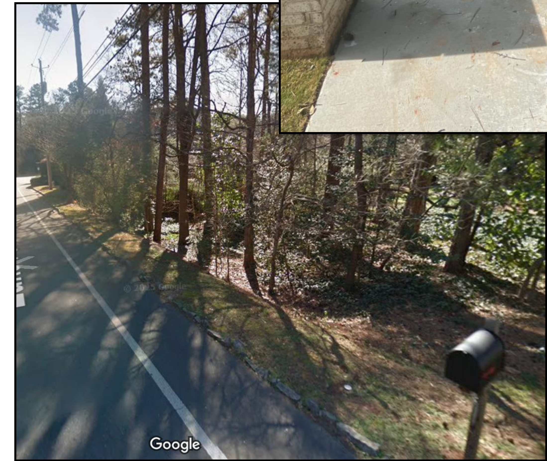
Before and after photos of S2185-1 Lake Forrest Drive Sidewalk Project currently under construction
