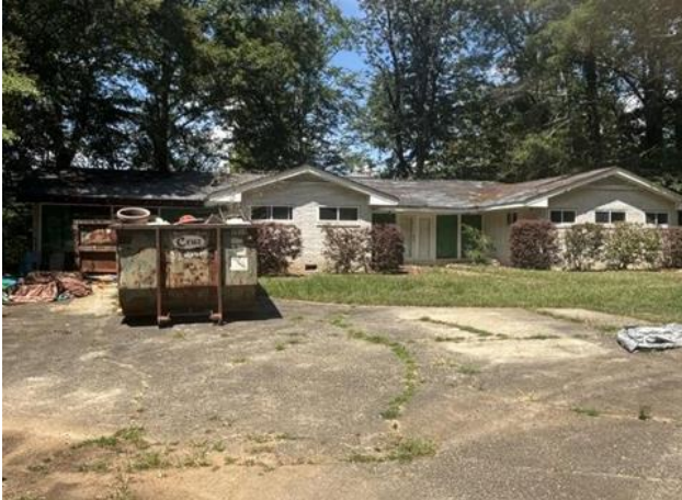
View of existing residential structure, facing North
