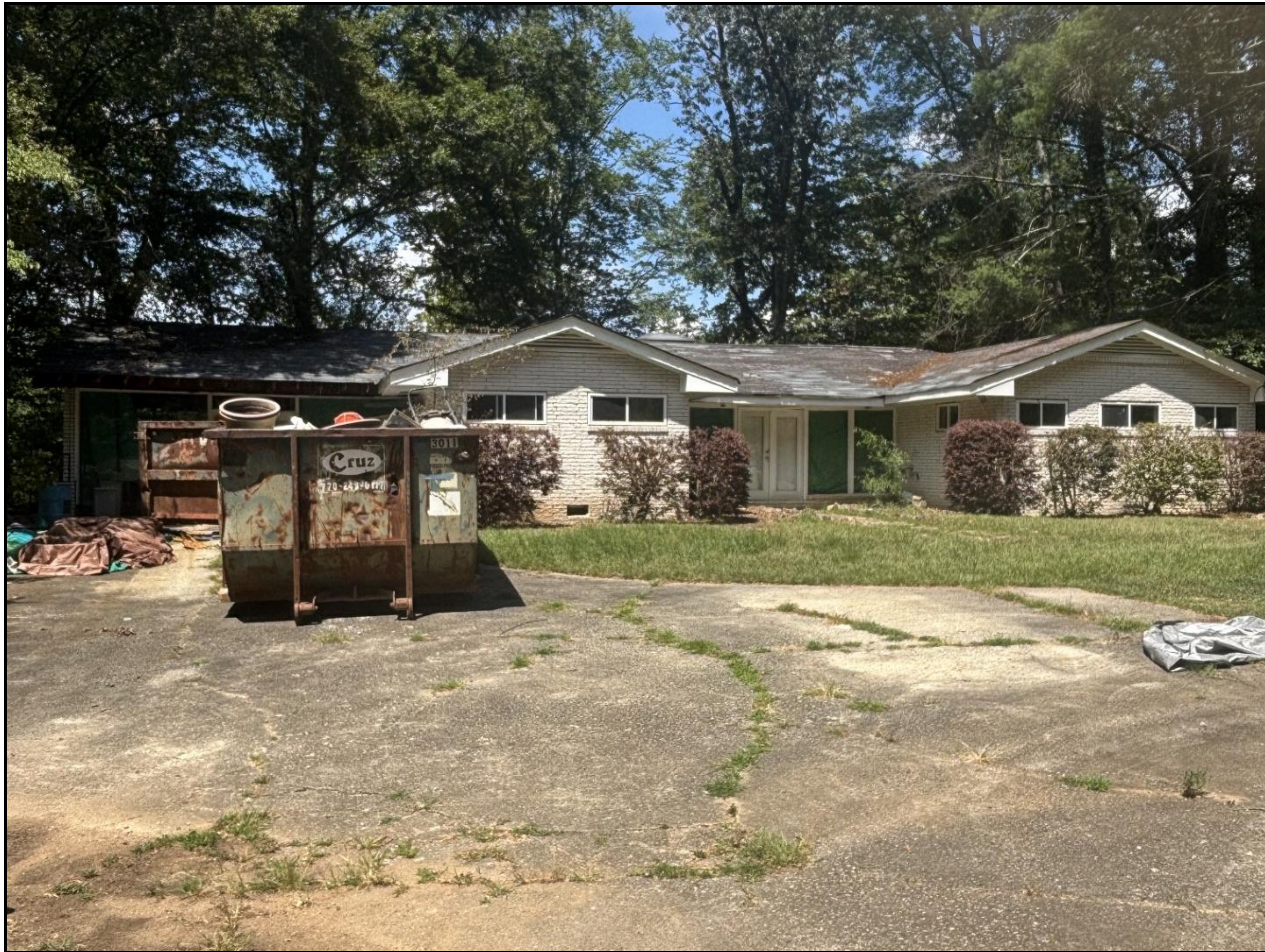
View of existing residential structure, facing North
