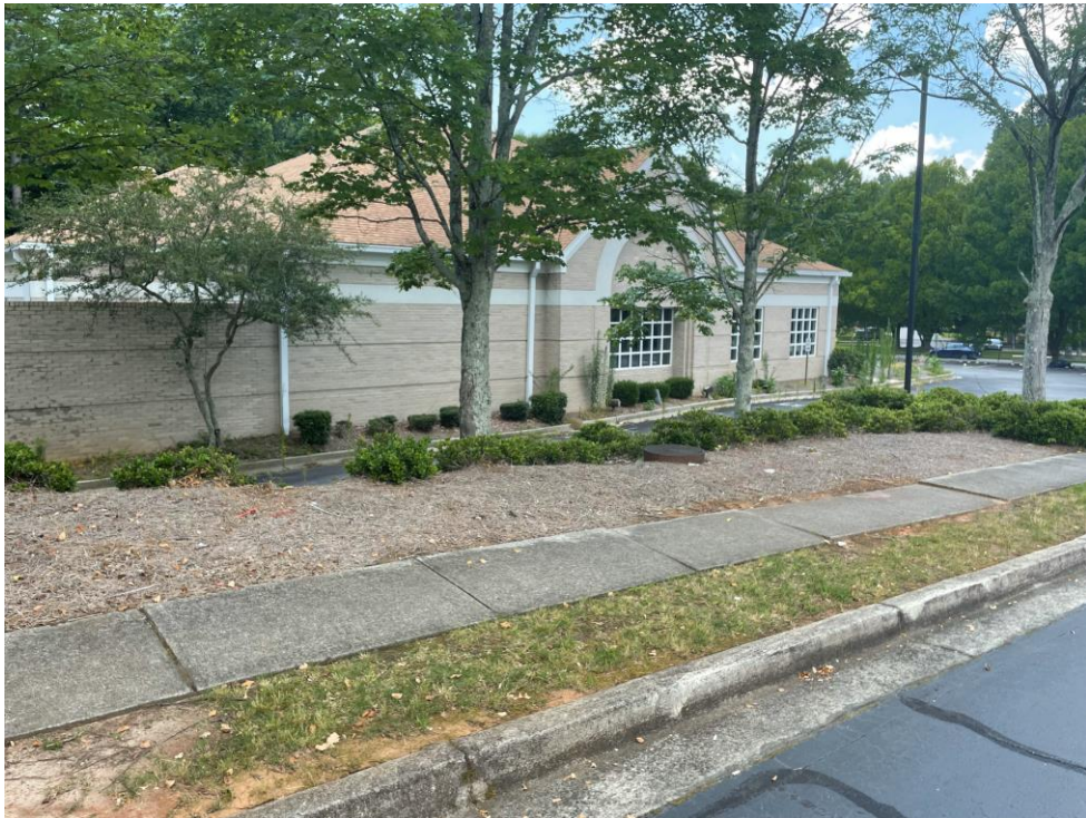
View of existing building and parking lot facing South
