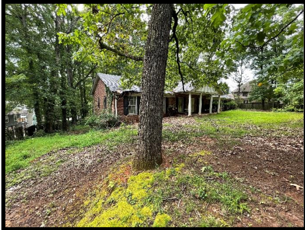
View of existing residential structure, facing southeast
