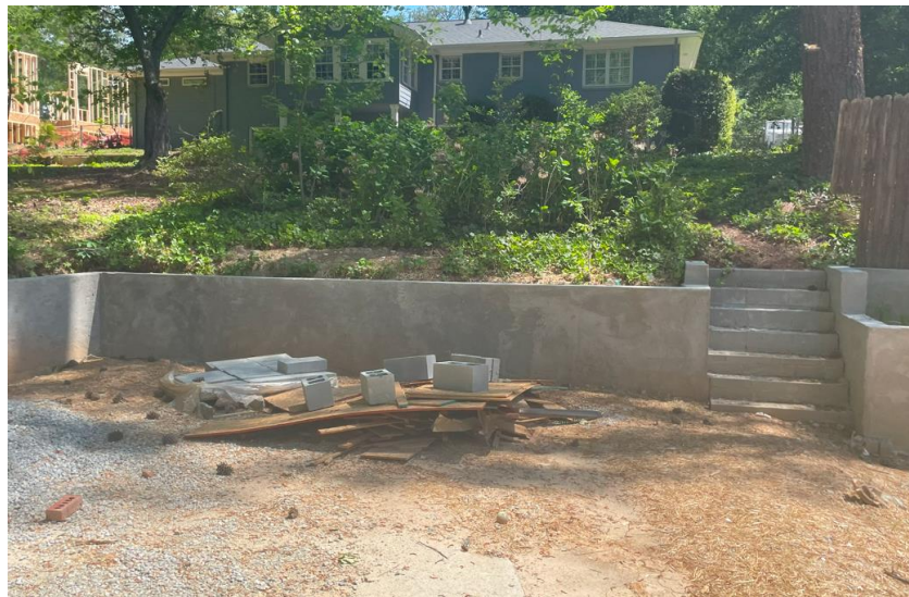
Rear of home facing east
