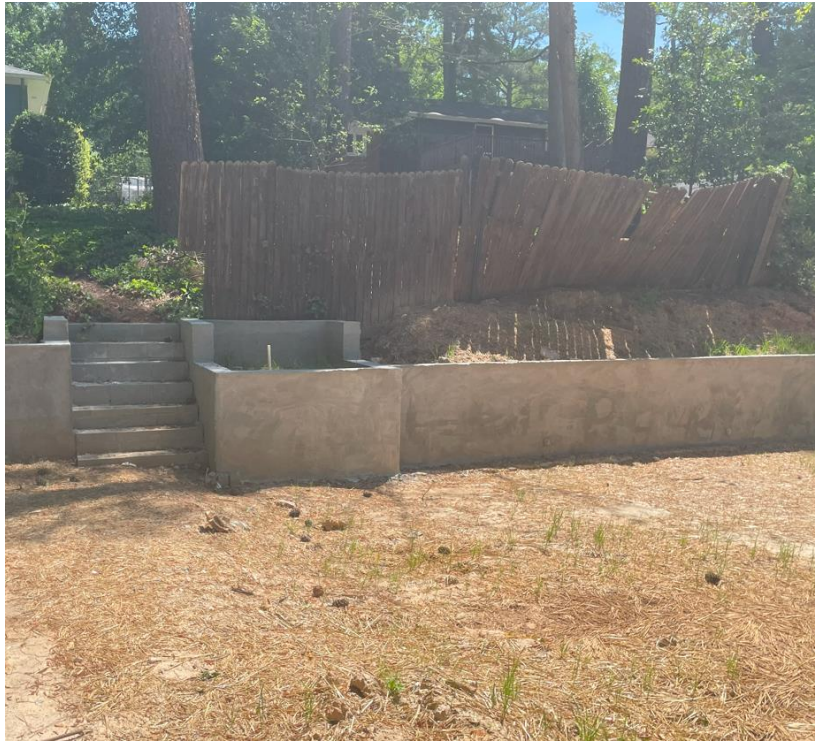
Rear of home facing east
