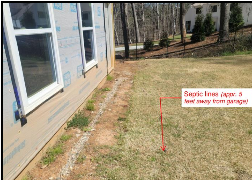
View of approximate septic line location
