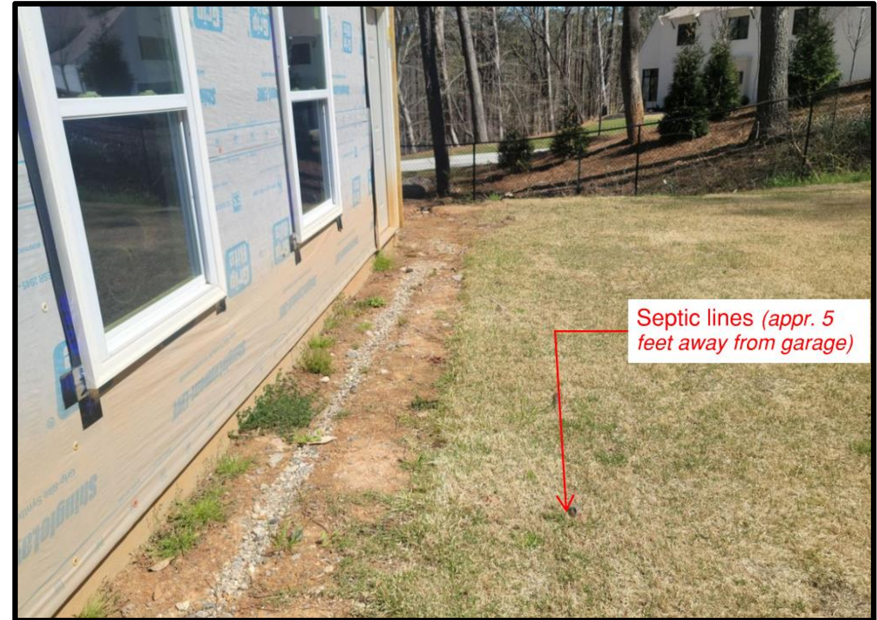
View of septic line from garage
