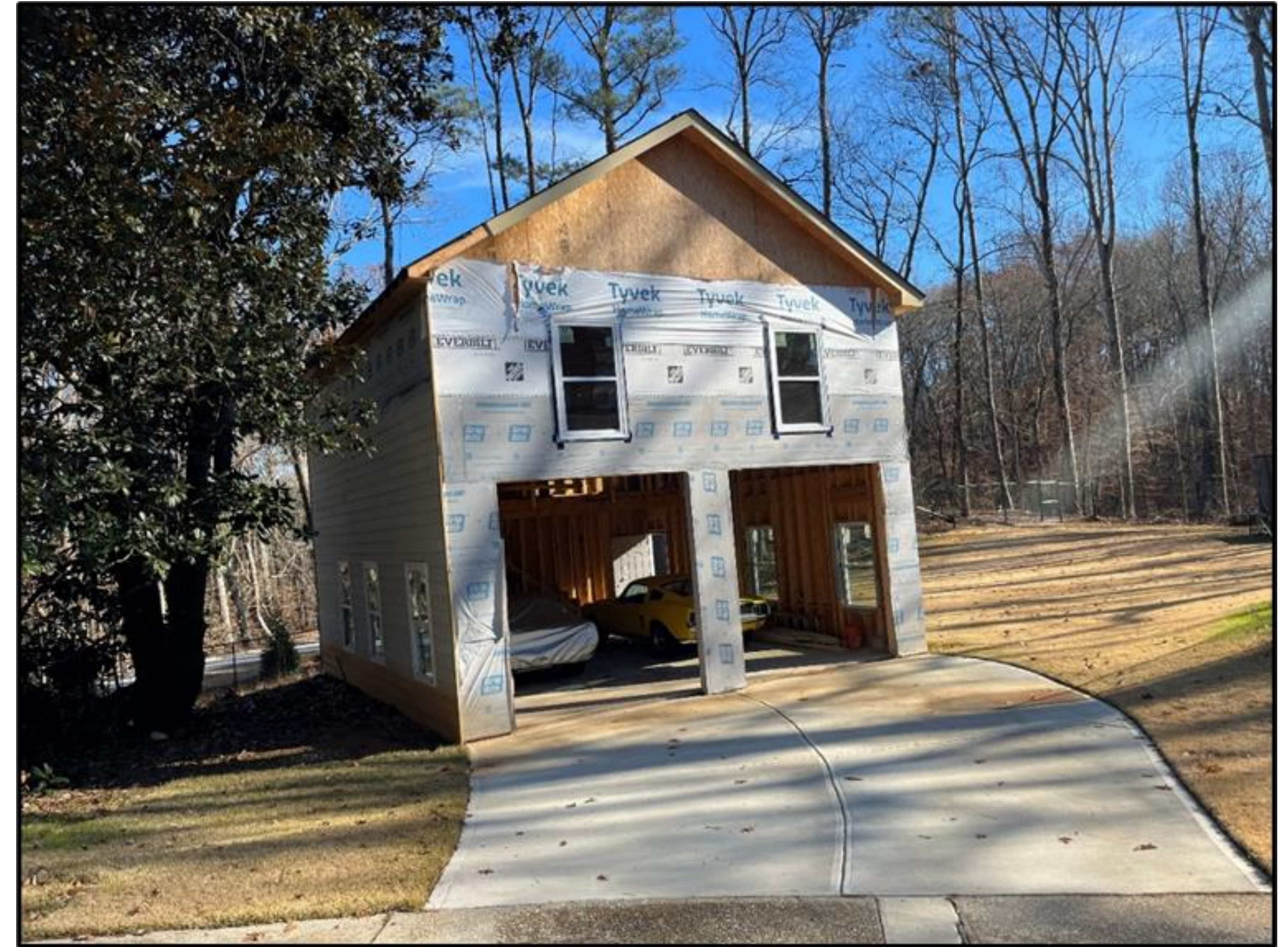
View of unpermitted garage on Skyridge Trail
