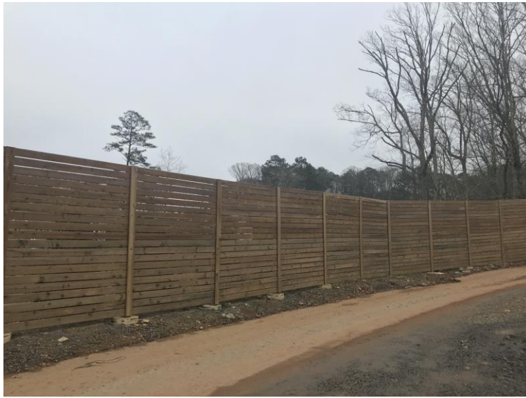
View of the existing fence by the maintenance area
