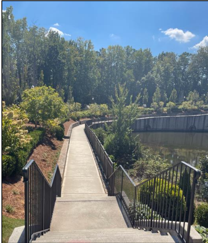
Existing sidewalk path that circumnavigates the pond/stormwater management facility.
