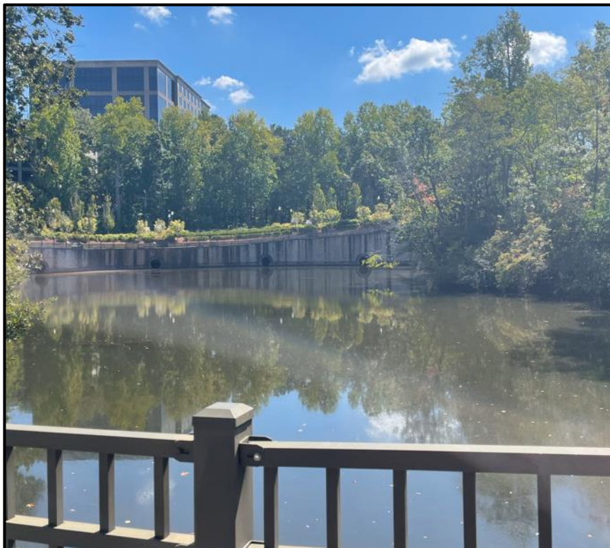
Image of existing pond/stormwater management facility, standing on Aria Boulevard
