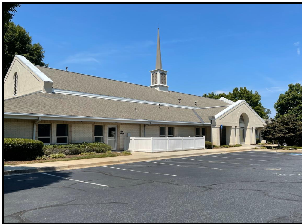
View facing northwest showing rear of meetinghouse
