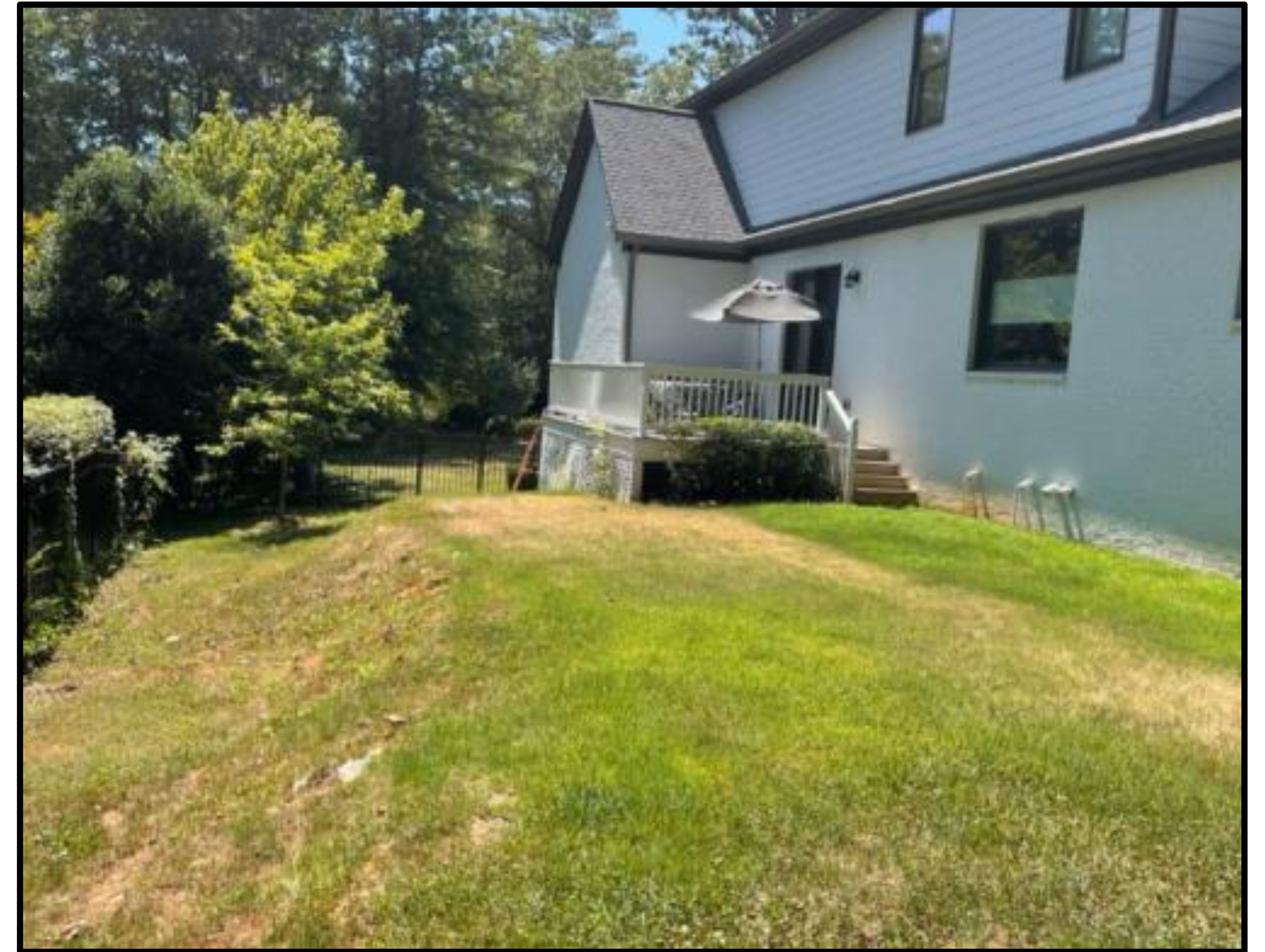
View facing west showing the existing Underground Water Quality Device and deck
