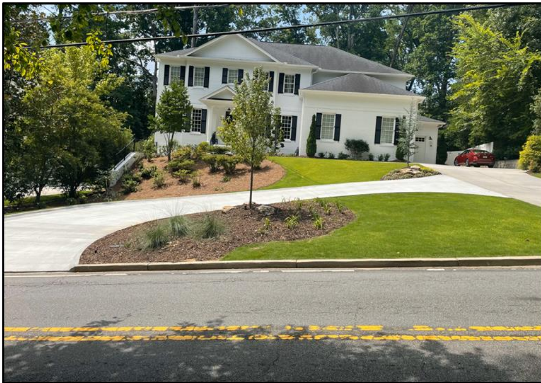
View of home and noncompliant driveway (to the left) standing on Franklin Road looking south
