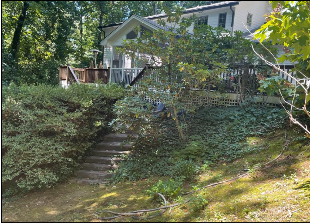
View facing north showing the rear of the home
