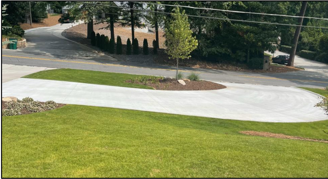
View of driveways facing north
