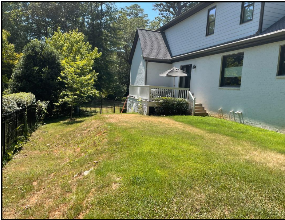
View of existing Unground Water Quality Device and deck
