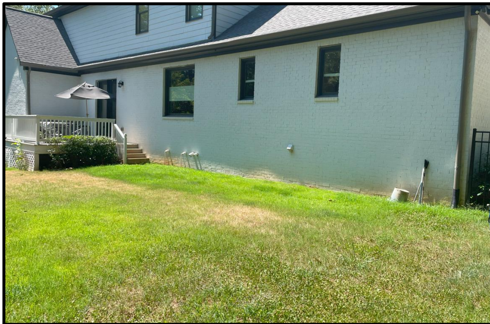
View facing west showing the existing Underground Water Quality Device and deck
