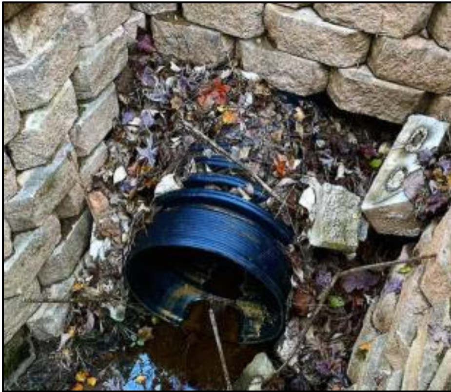
View of extended pipe and retaining wall in the 25' State Water Buffer
