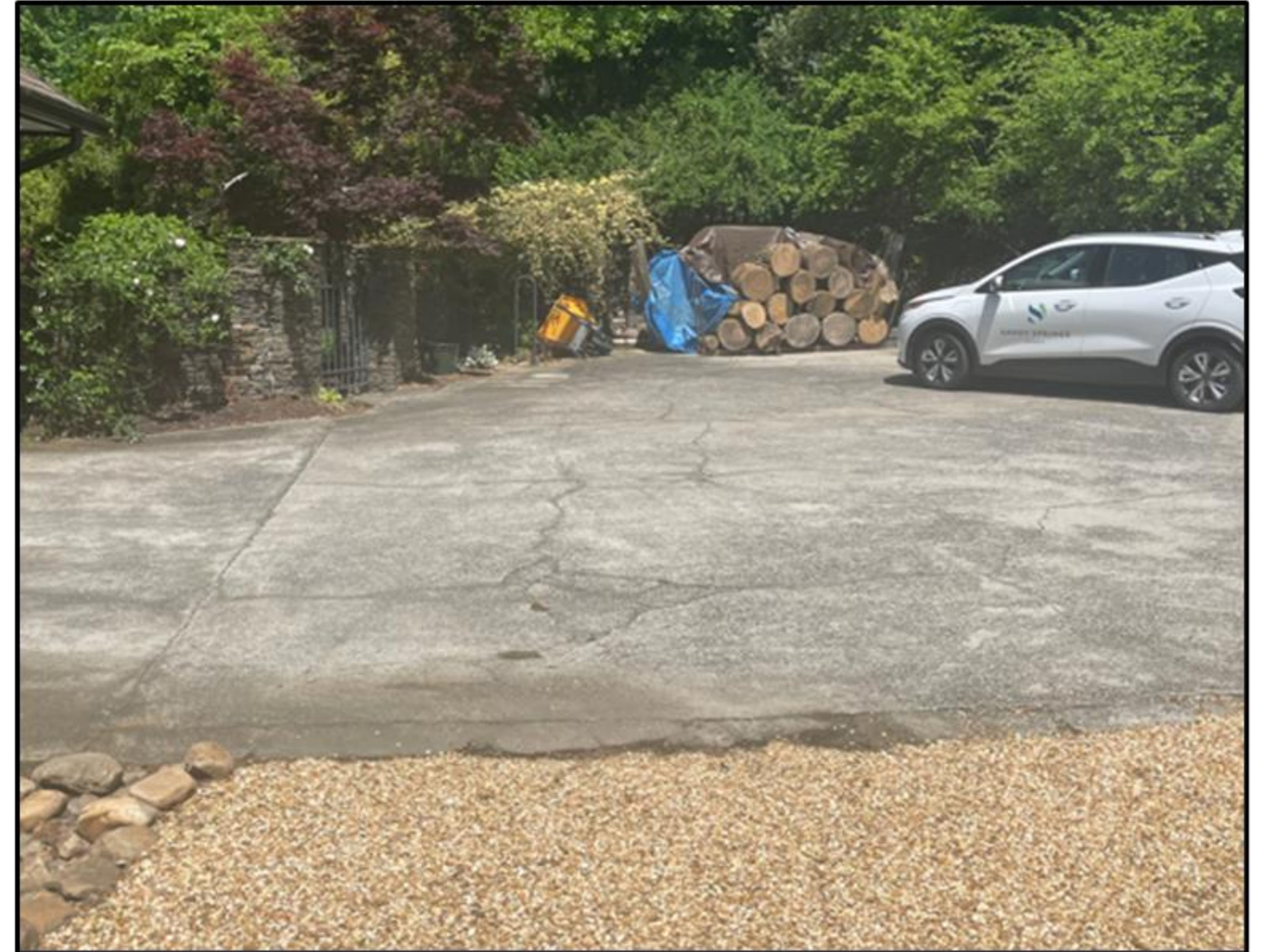
View of driveway from side property line looking towards the pool
