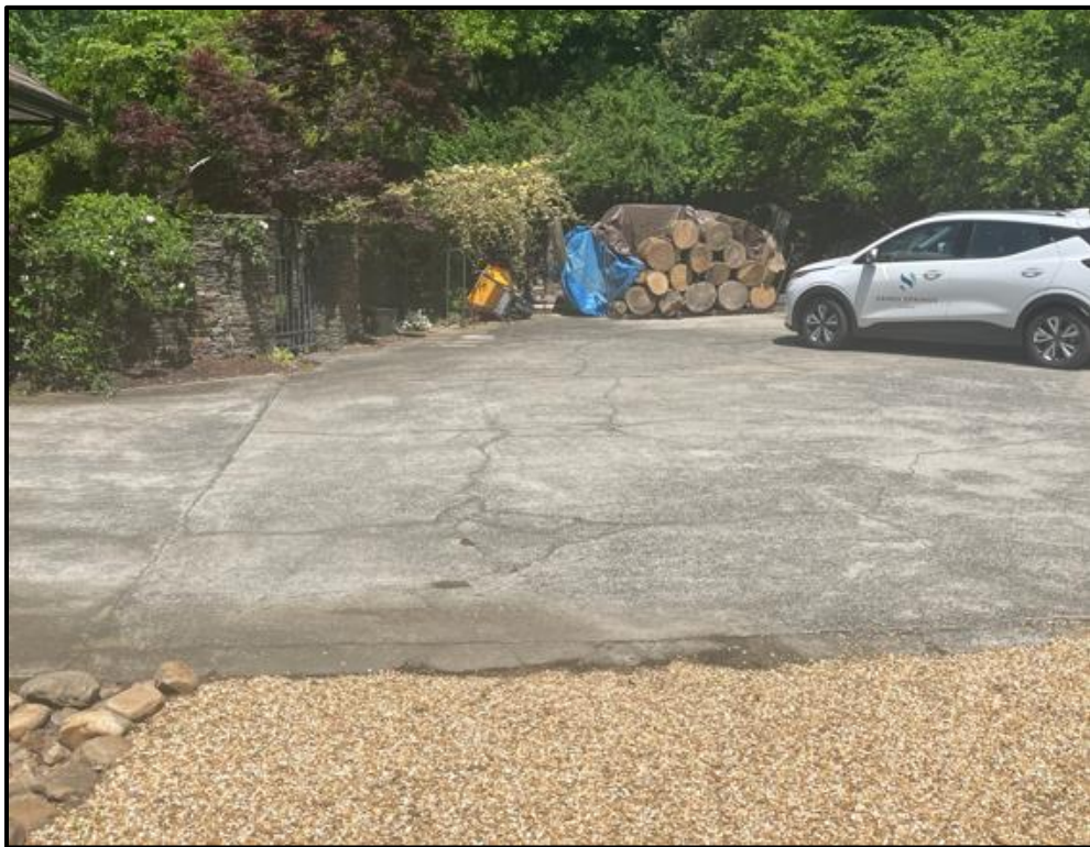
View of driveway from side property line looking towards the pool
