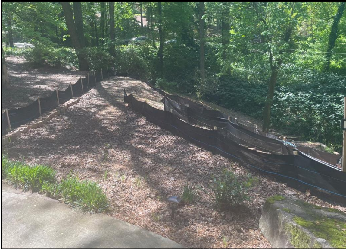
View standing near home on driveway facing south towards River Valley Road
