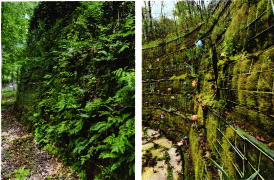
Examples of Living/Earthen Walls
