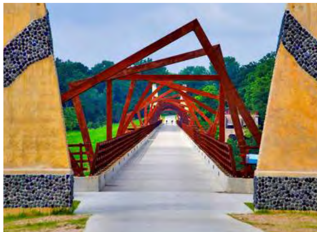
LEFT: The High Trestle Bridge, Woodward, IA
