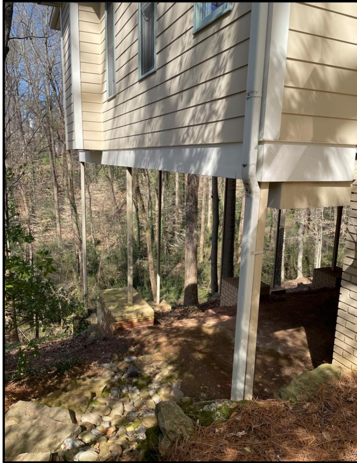
View of existing piers facing rear of home
