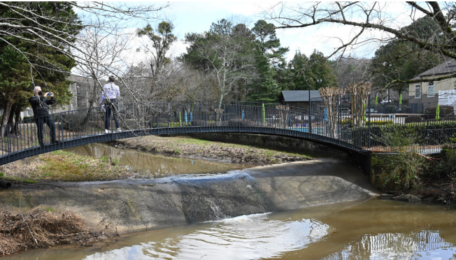
A dam/embankment across Long Island Creek
