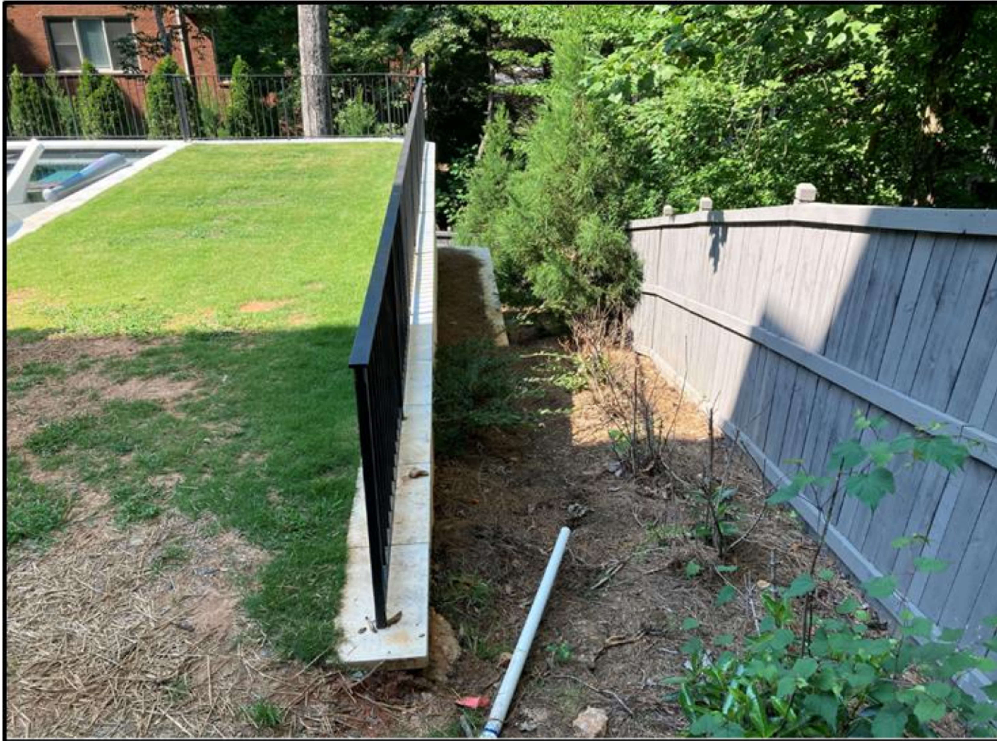
View of the tiered retaining walls looking north at the east property line
