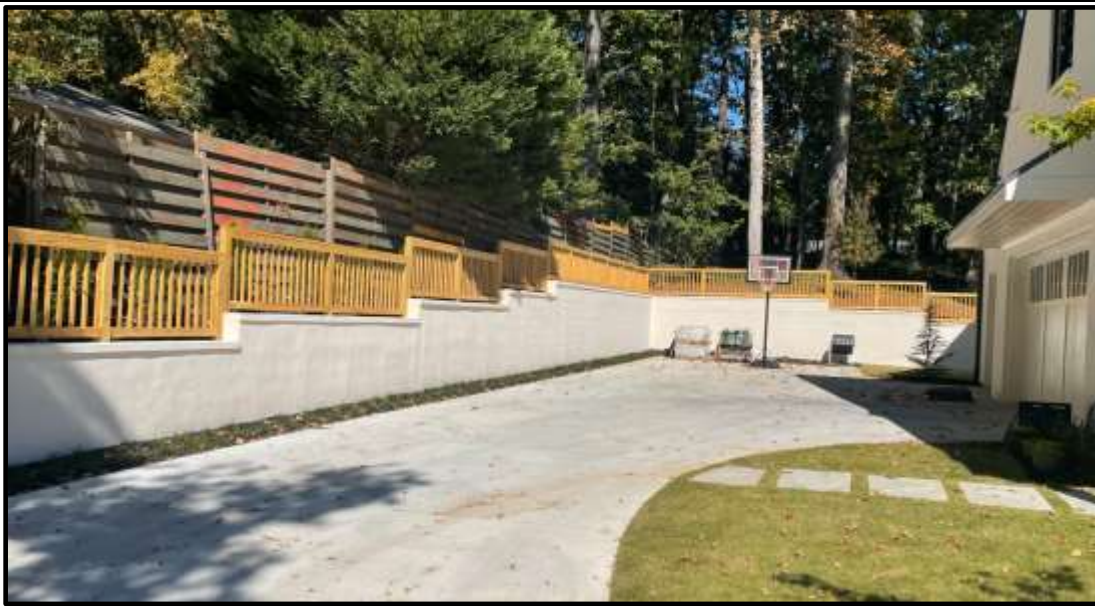
View looking north of the retaining wall to the west
