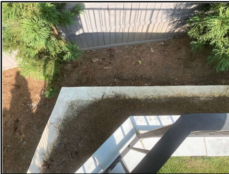
Aerial image of the angled portion of the retaining walls
