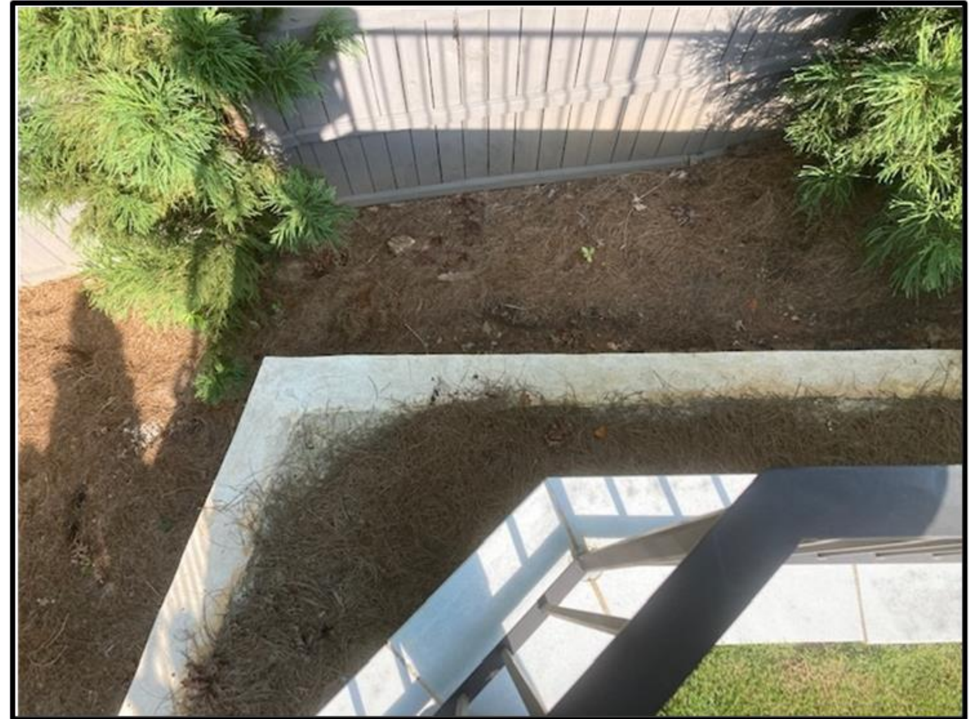
Aerial image of the angled portion of the retaining walls
