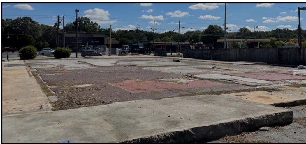
Image of the existing condition of the property looking east toward Roswell Road
