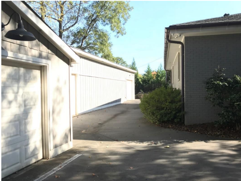
View to the rear of the existing primary structure and of the detached garage and warehouse structures
