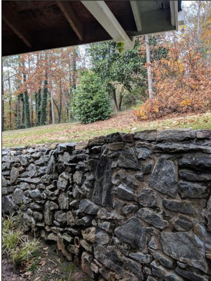
Existing retaining wall:
