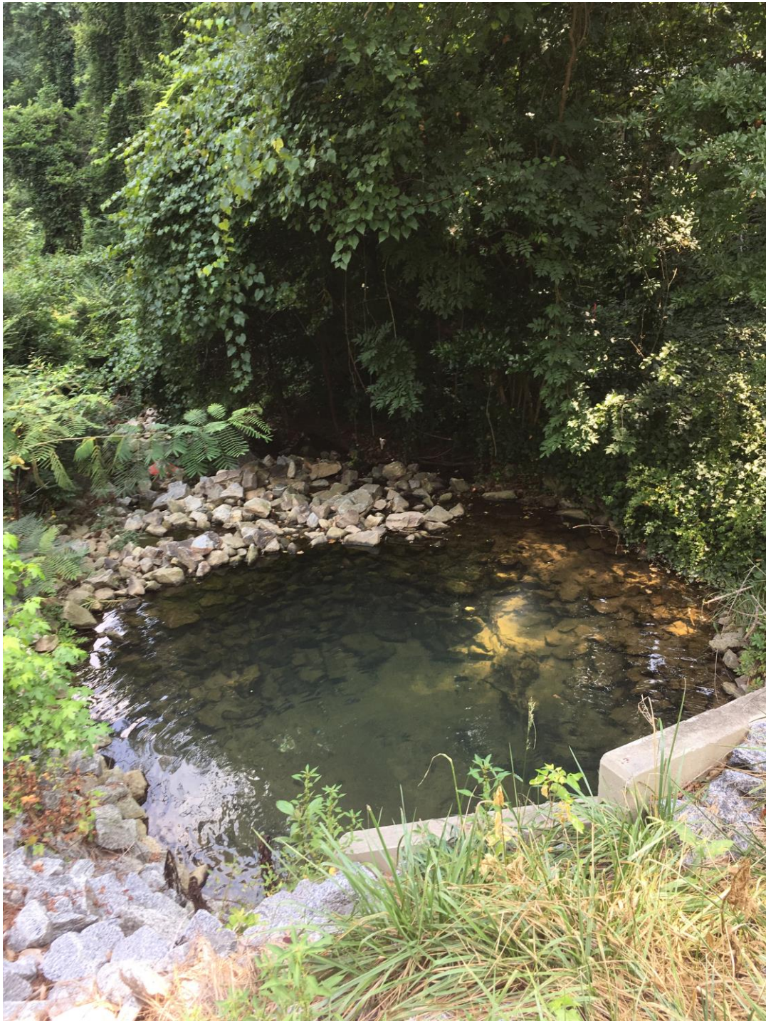
The stream and surrounding vegetation and culvert; view south from the Windsor Parkway sidewalk
