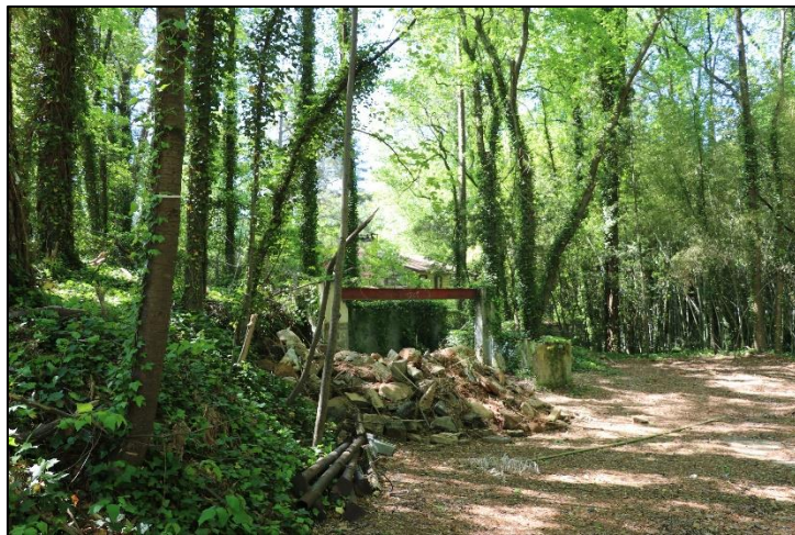
Piles of debris on site
