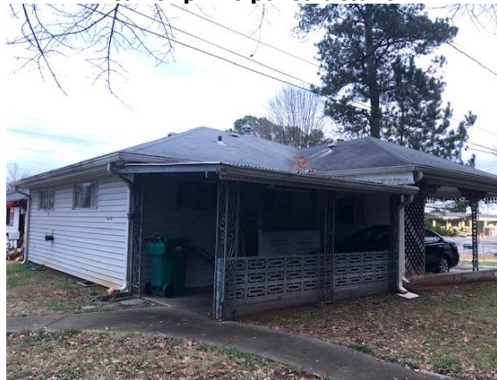
Rear of principal structure
