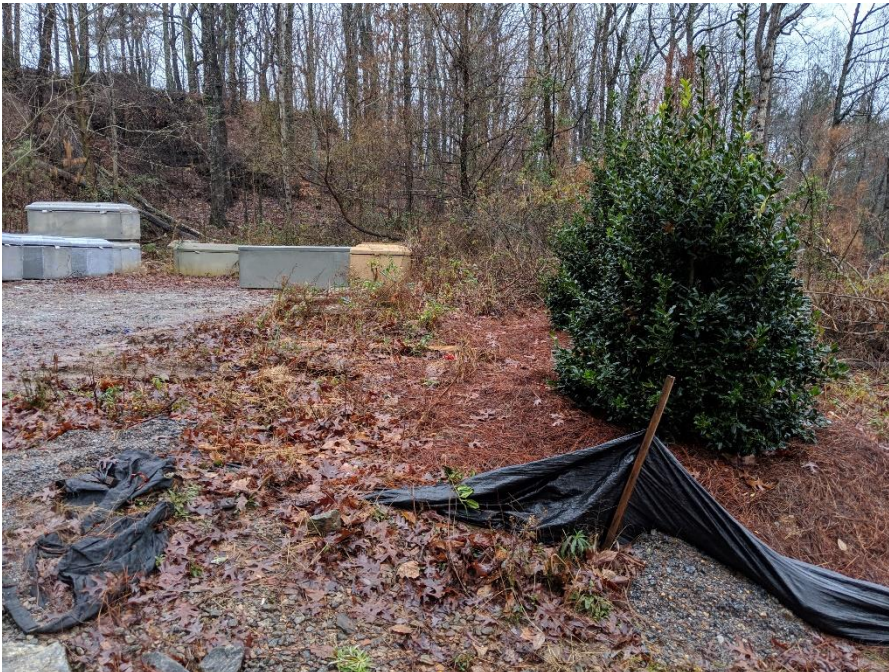
Side view of proposed fence installation location.
