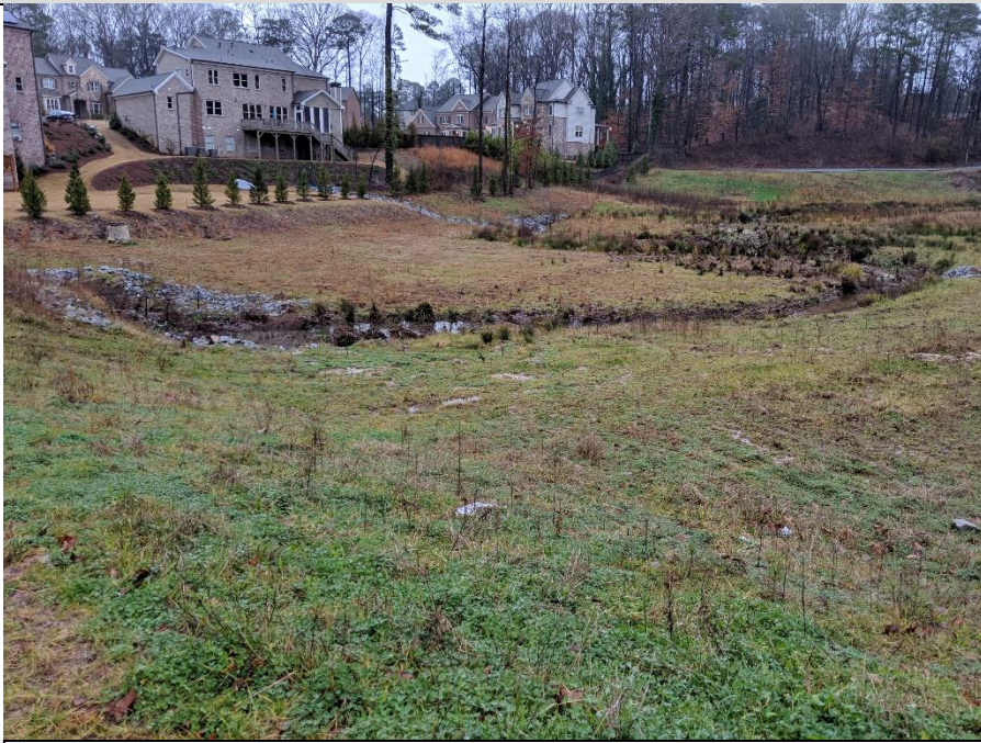
View of detention pond that was restored.
