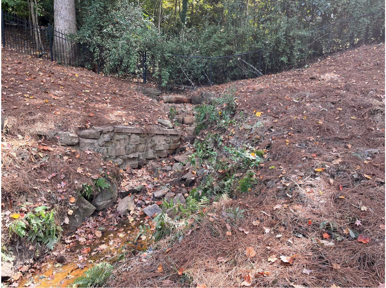
View of stream looking from pipe and wall to property line fence
