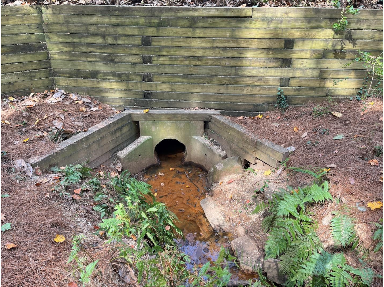
View of uphill side of pipe & wall
