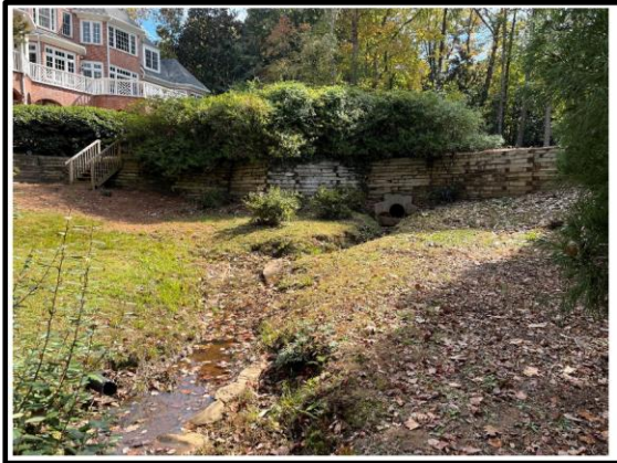
View of the downhill side of the pipe
