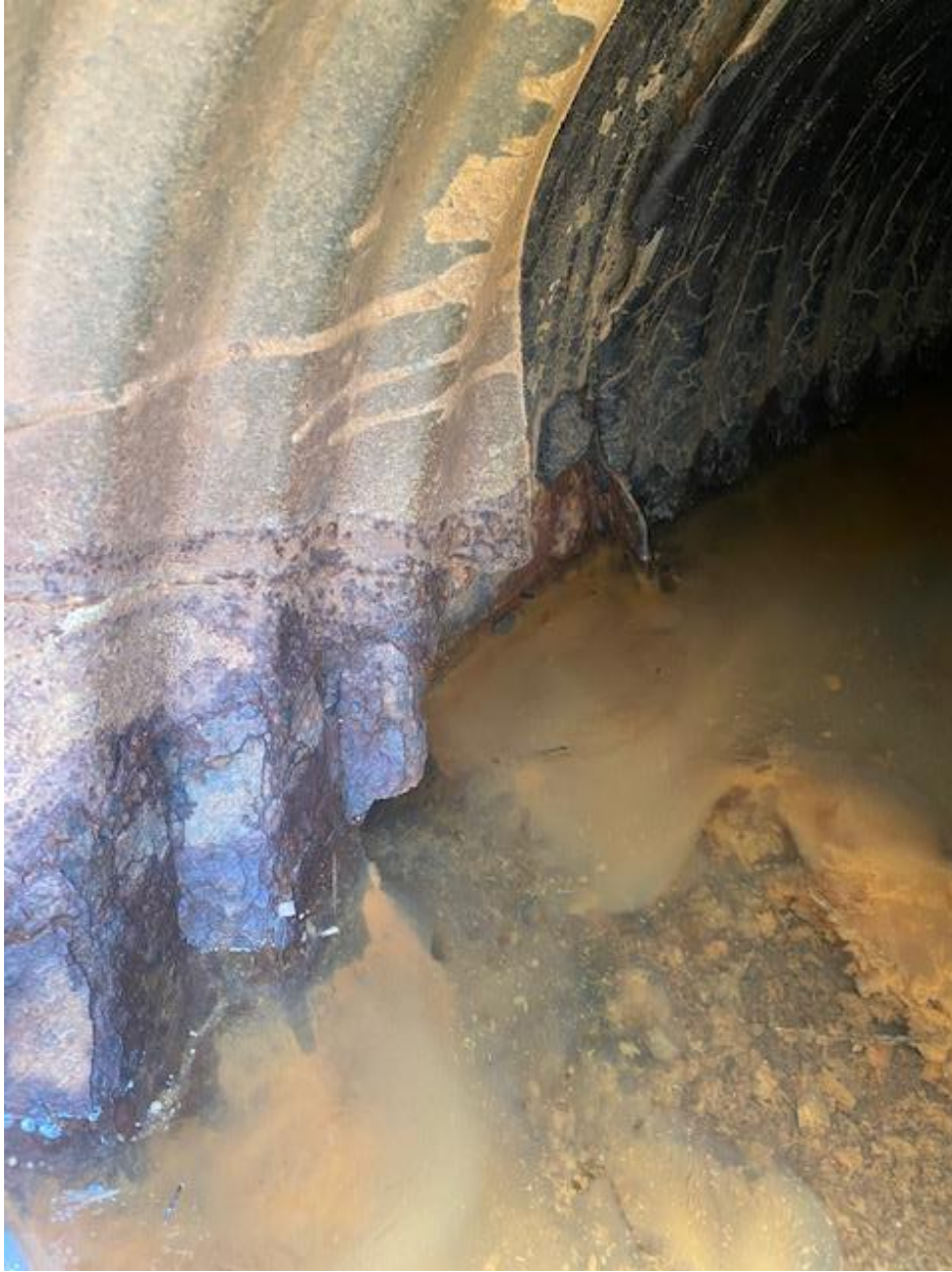
Upstream side of pipe
