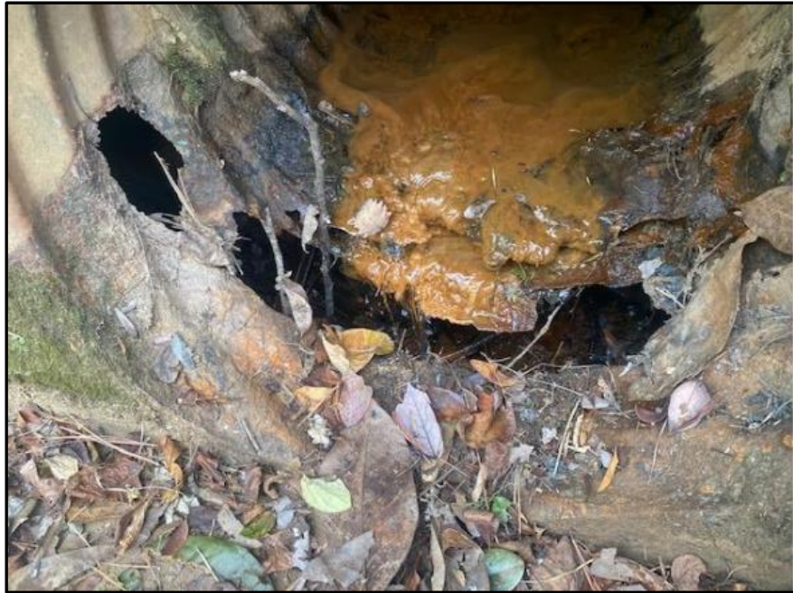
View of downhill side of the pipe
