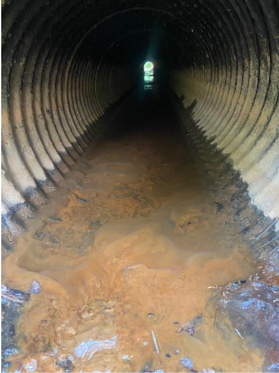
Downstream side of pipe
