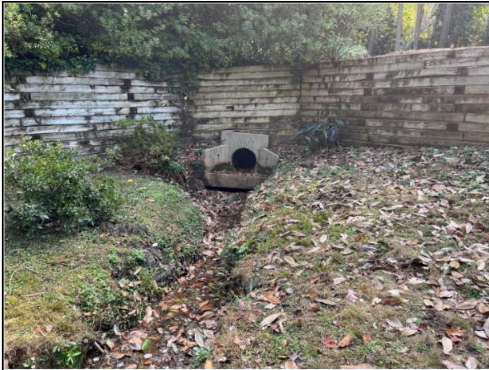
View of downhill side of pipe
