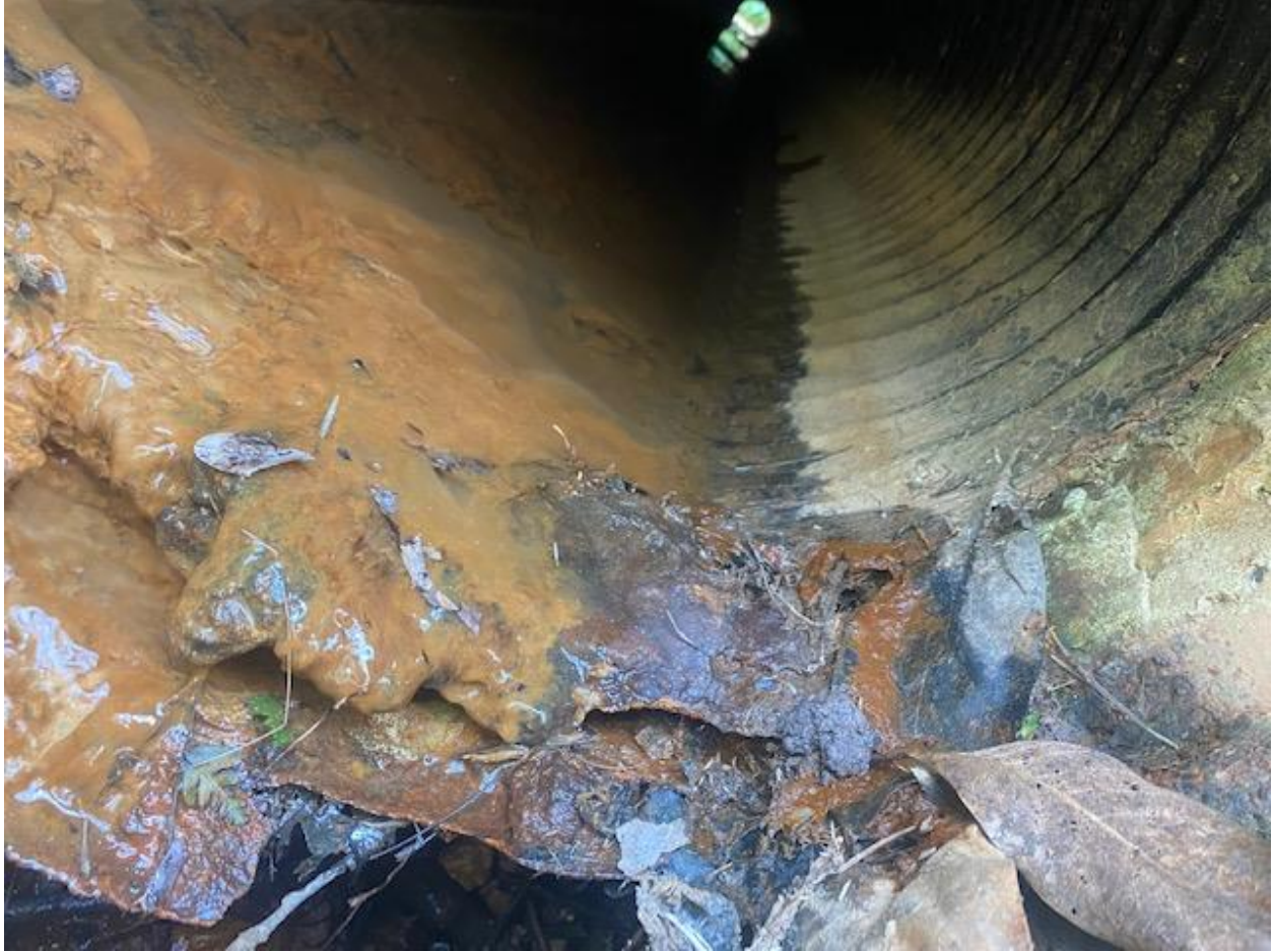
Downstream side of pipe
