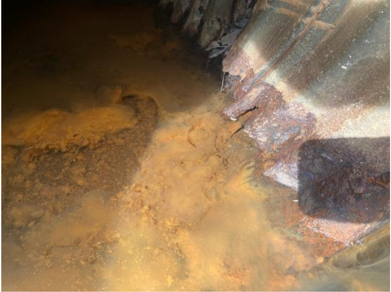
Upstream side of pipe
