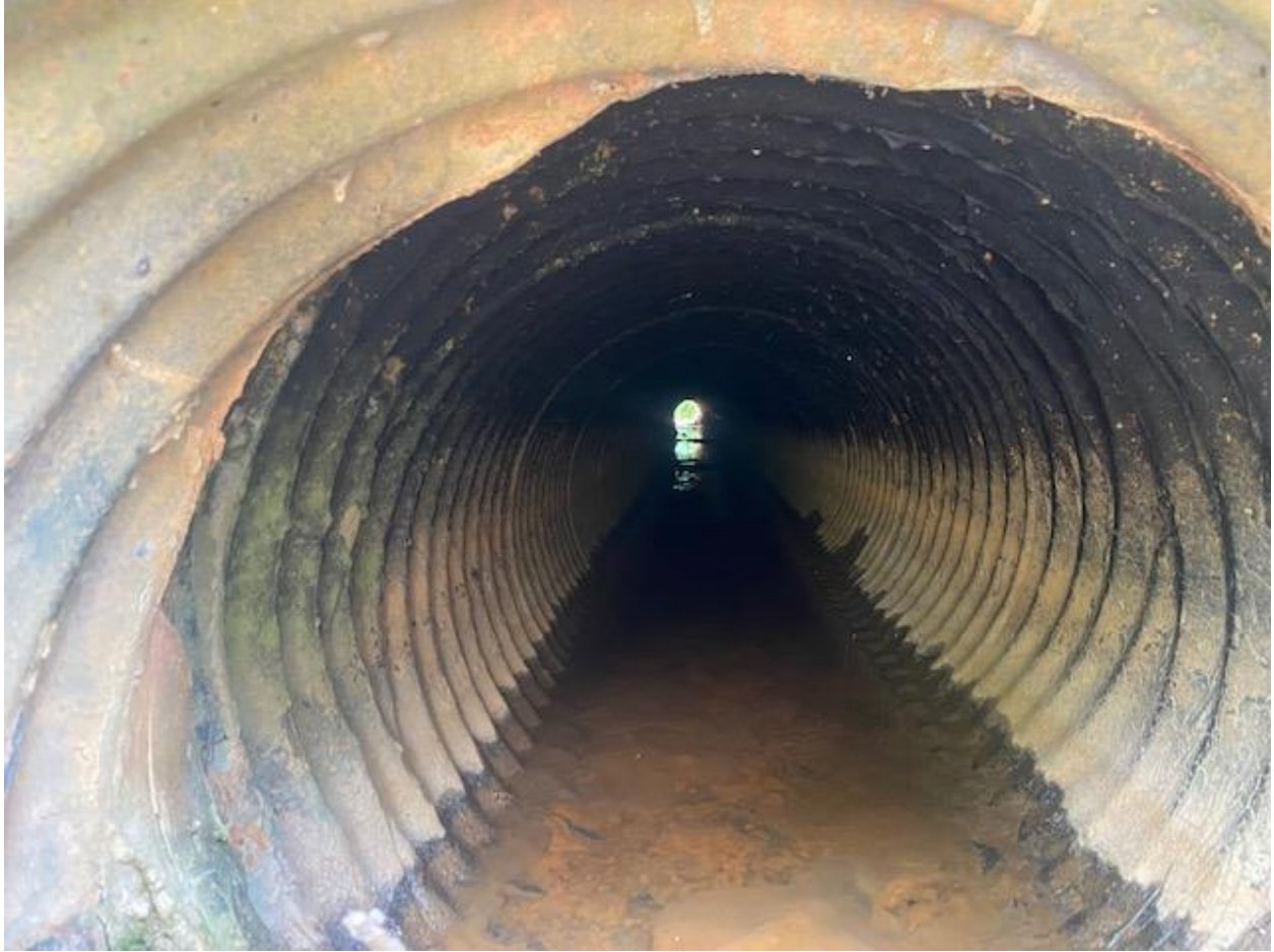
Downstream side of pipe
