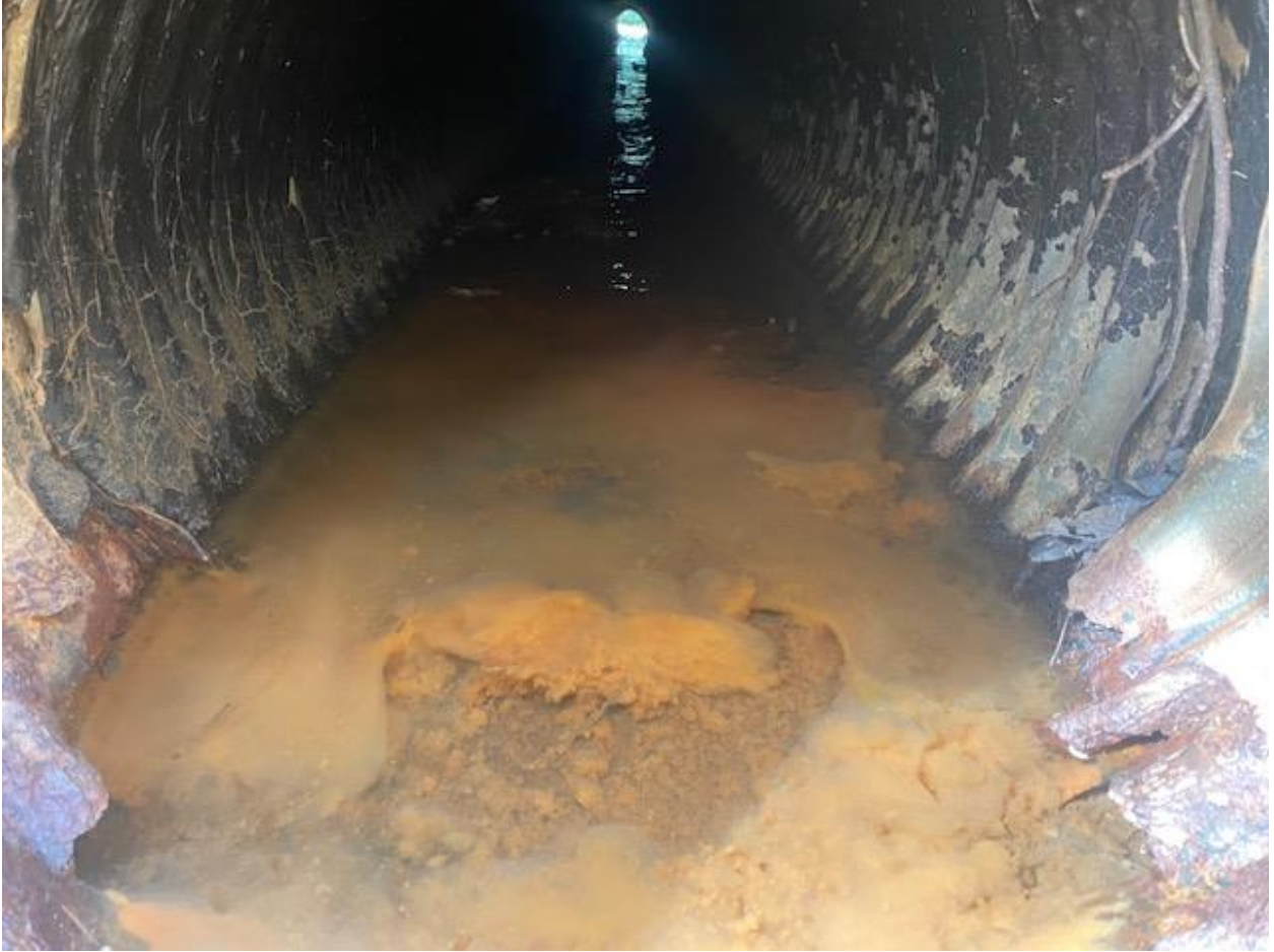
Upstream side of pipe
