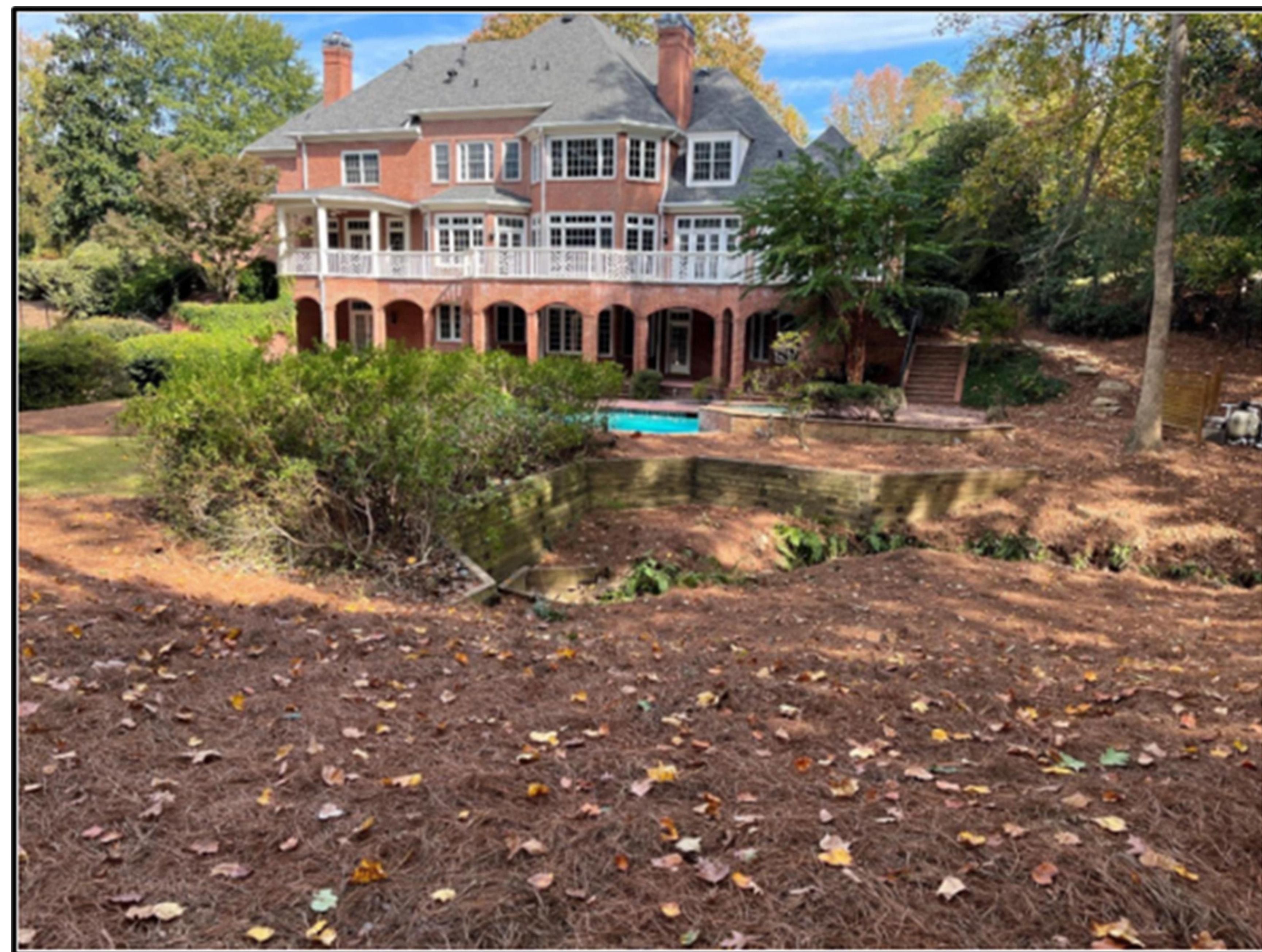
View looking north from the rear yard
