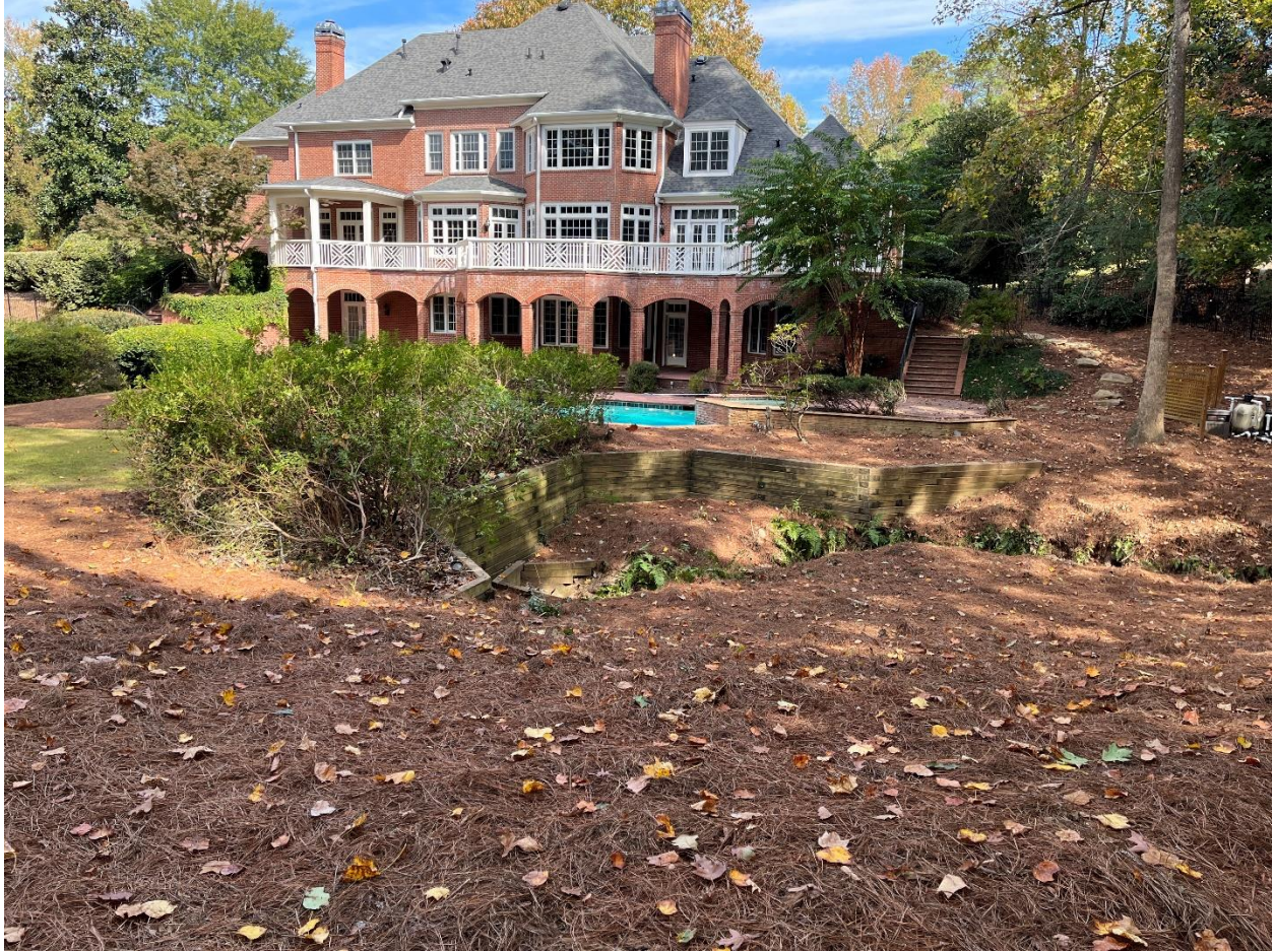
View of back of house with uphill side of stream on left with ex wood walls
