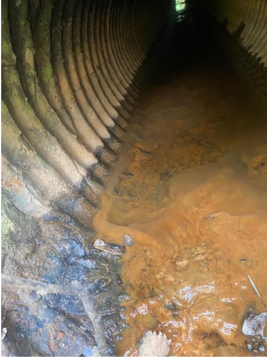
Downstream side of pipe
