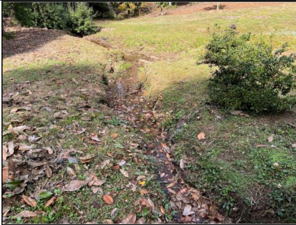
View of stream facing downhill side of pipe
