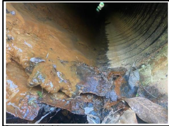
View of the downstream side of the pipe
