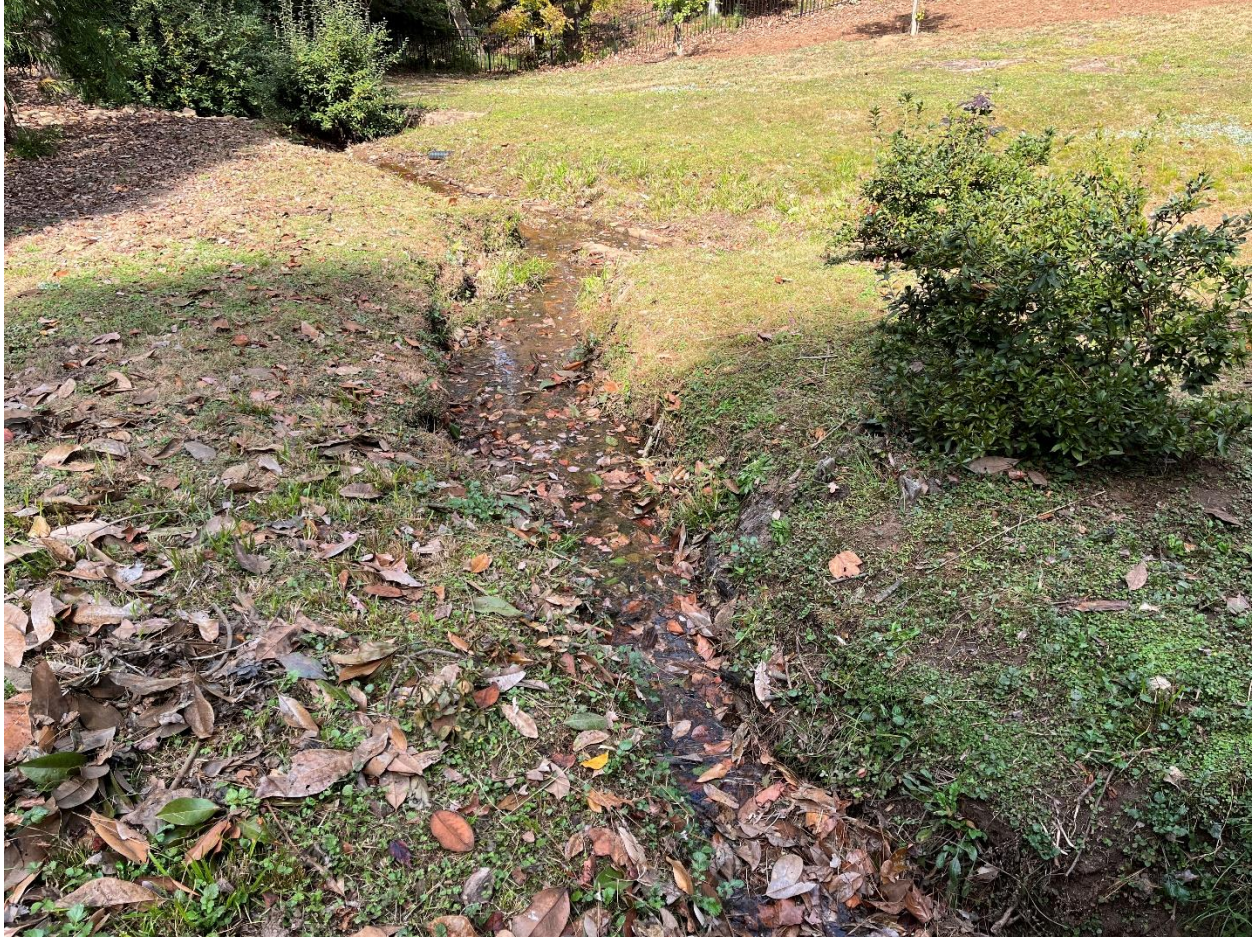
View of stream looking from downhill side of pipe
