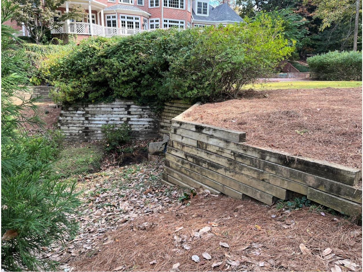
View of downhill side of pipe & wall
