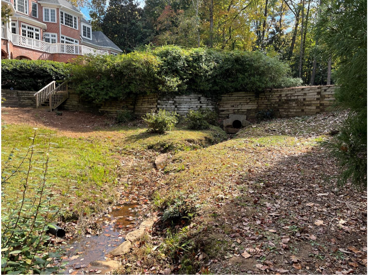
View of wood walls and downhill side of pipe
