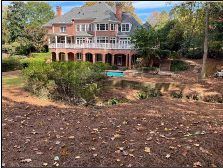
View looking north from the rear yard
