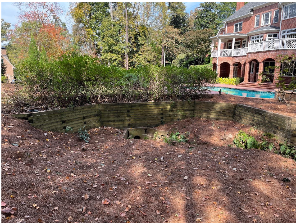
Uphill side of stream wood walls
