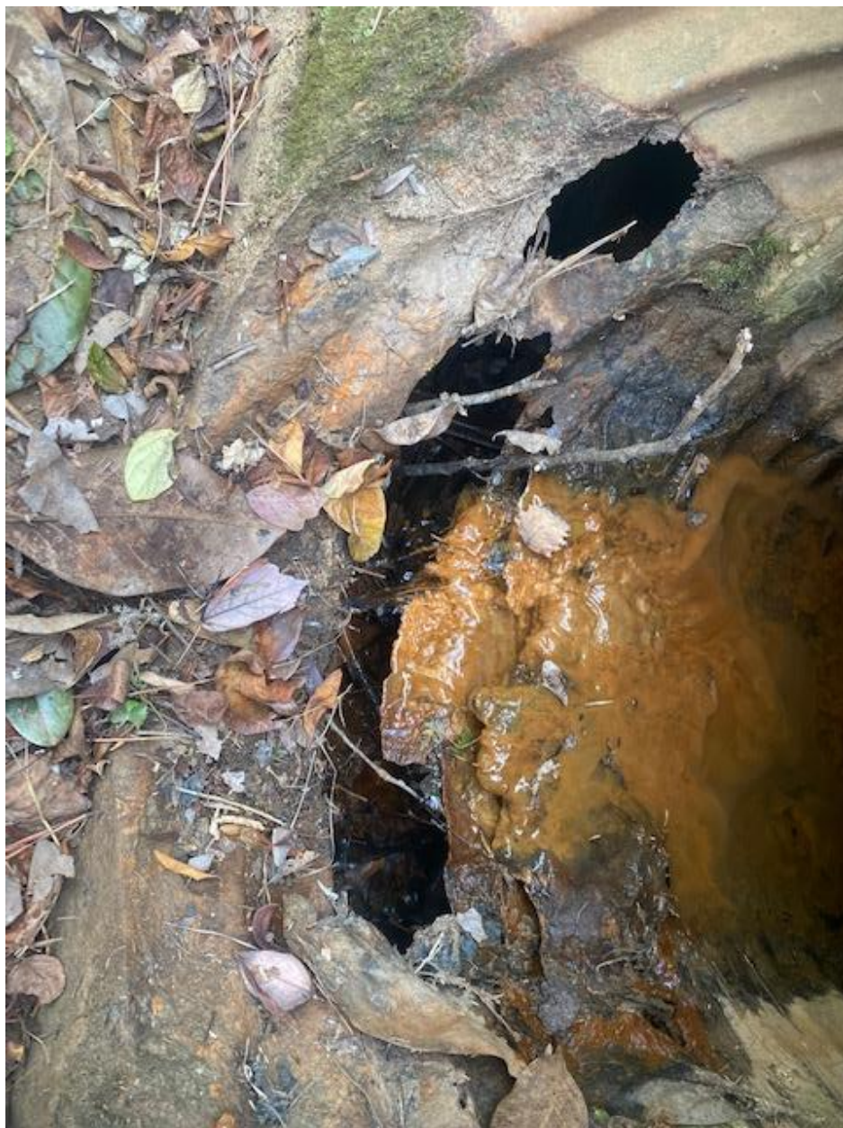
Downstream side of pipe
