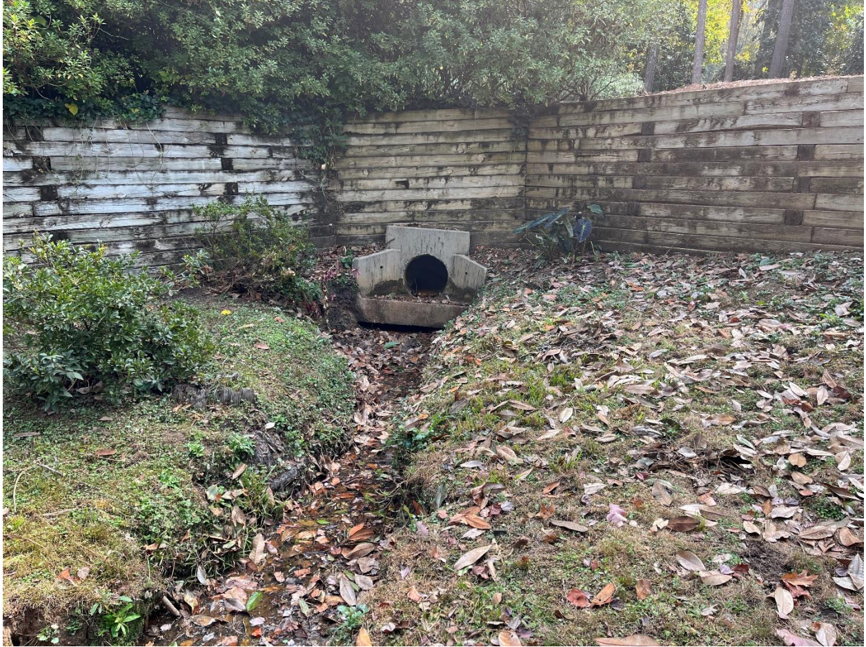
View of Downhill side of pipe
