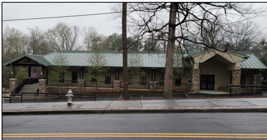
Facing west on Blue Stone Road, viewing the front of the Heritage Building
