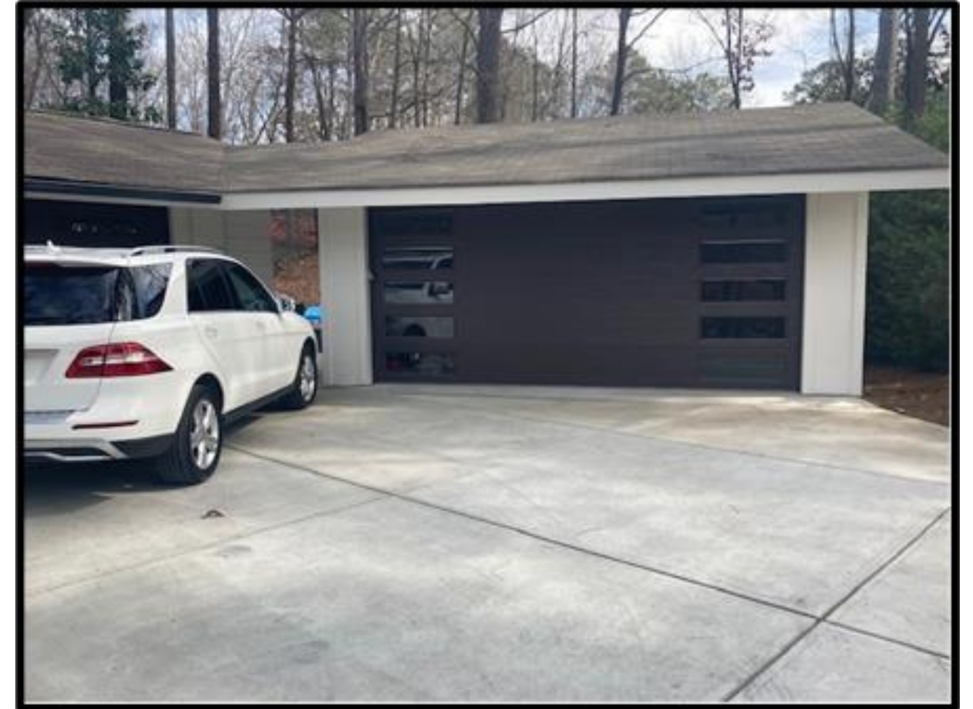
View of existing garage within the setback
