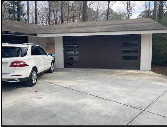
Existing garage within the setback
