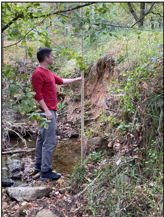
P-2 VERTICAL 6 FOOT BANKS WITH ON-GOING EROSION
