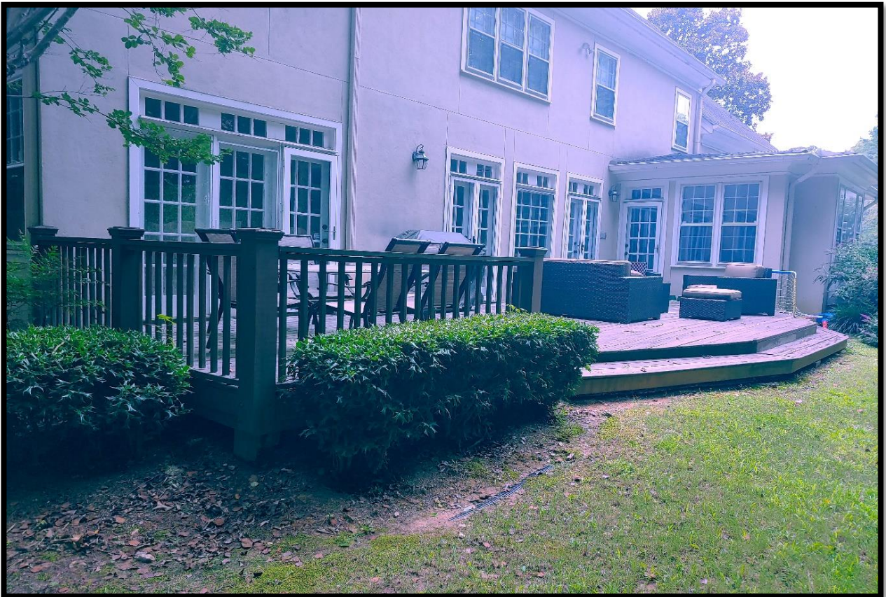
Above: The uncovered deck in the rear yard of 55 Wembley Lane.
