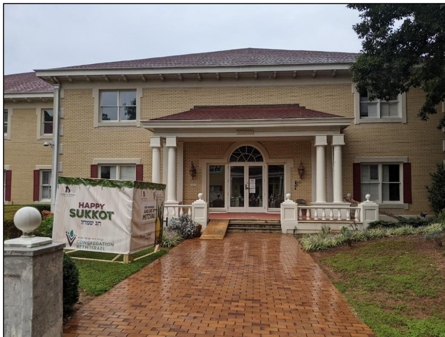
View facing north of side (main) entrance into the school from entry drive
