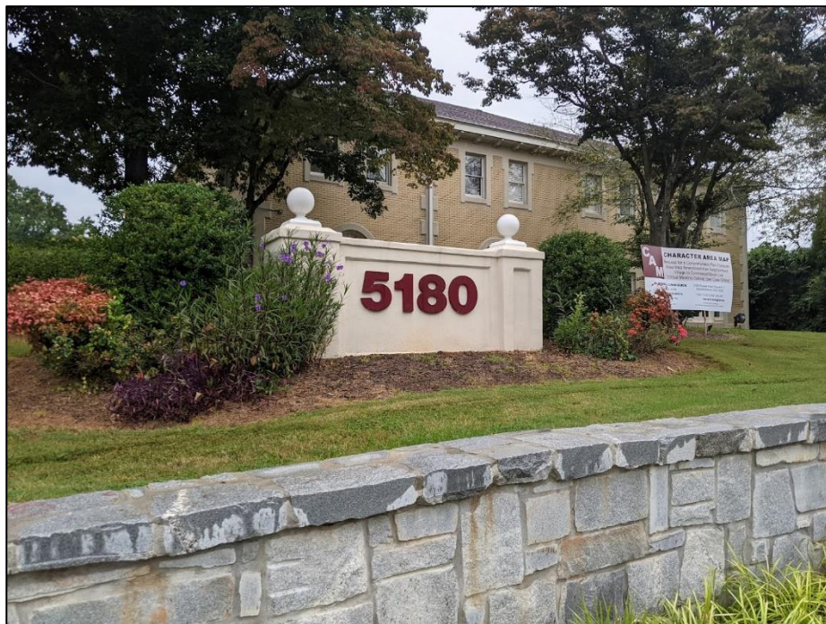
View facing northwest, with the subject property directly in view
