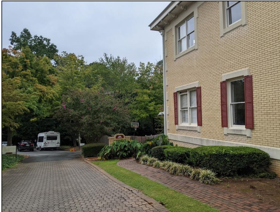
View facing west, showing the building and the rear of the property in the distance
