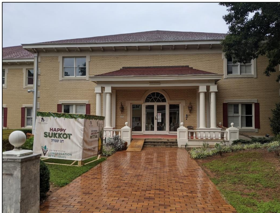
View facing north of side (main) entrance into the school from entry drive
