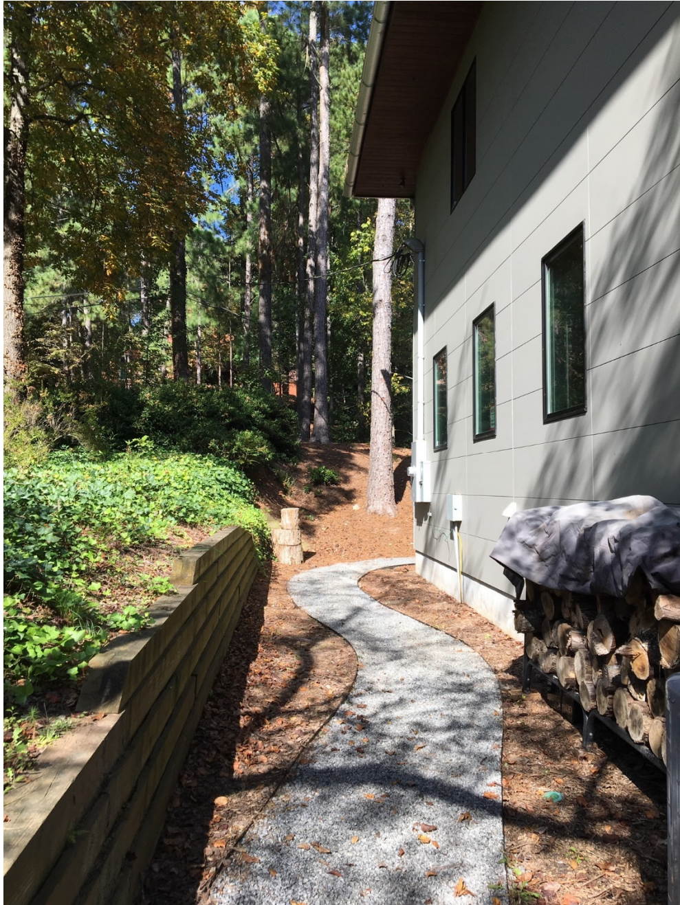
West side of home, generator location
