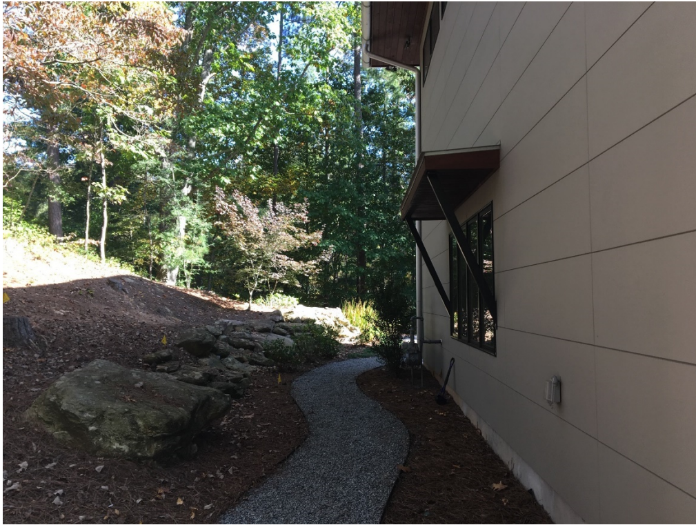
East side of home, front of house (location of utilities)
