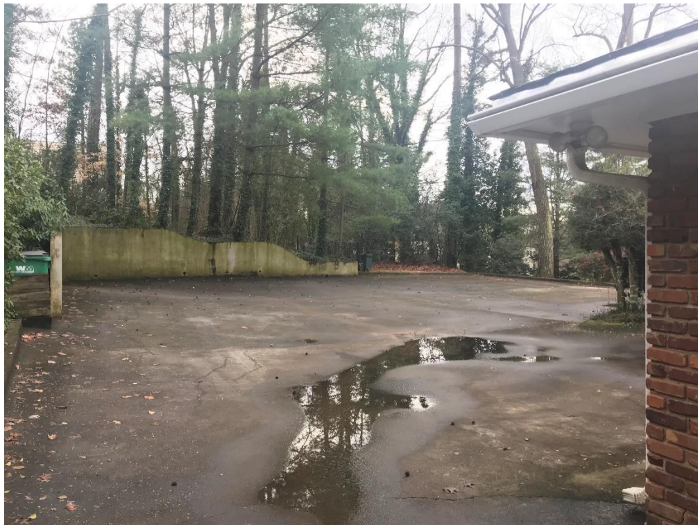
View of rear of 145 Cliftwood Drive
