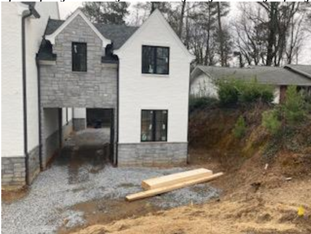
View of home facing east showing the south side grading cut to the right of the garage
