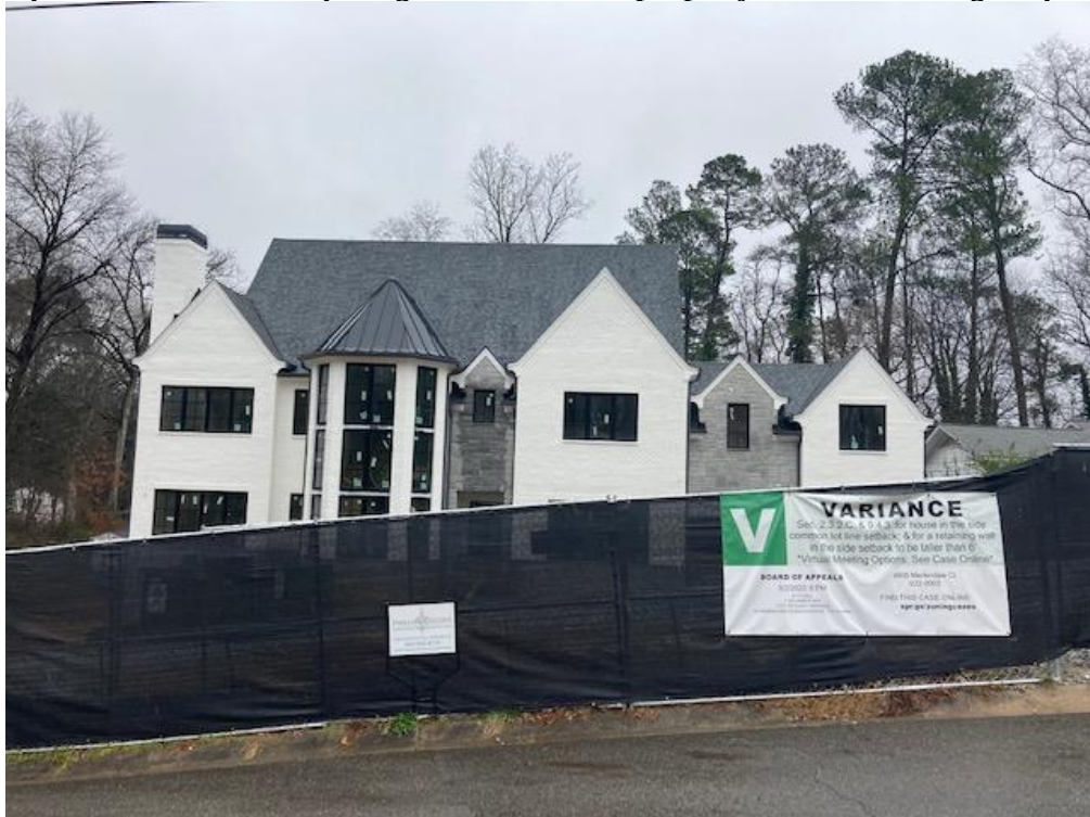
View from Merlendale Ct facing east, the south property line is to the right of house
