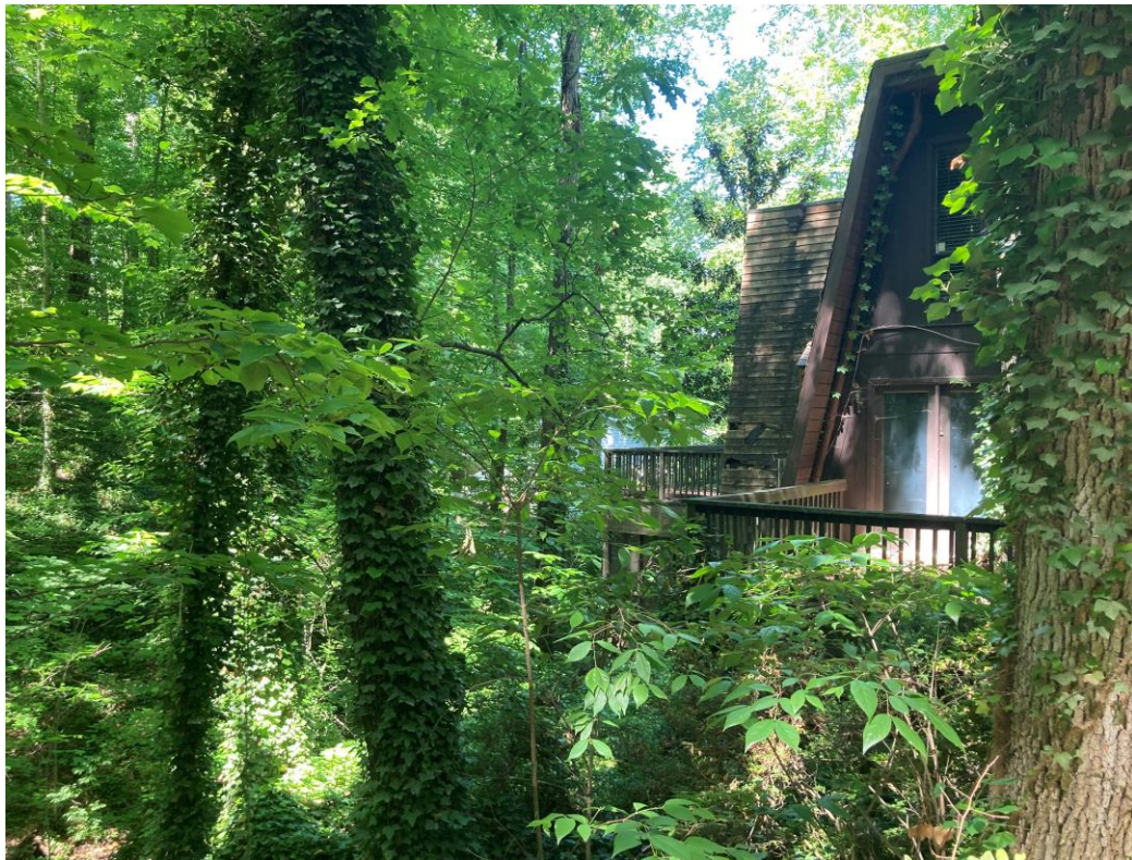
Decks on south side of residence
