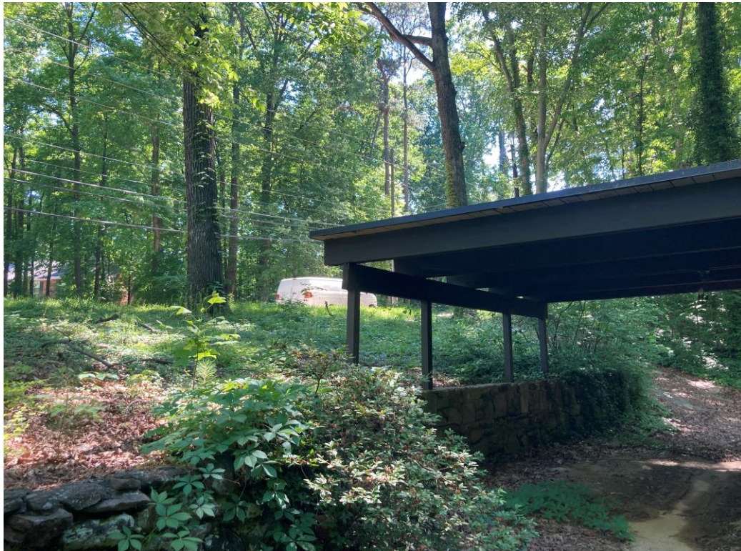
Carport and view northeast
