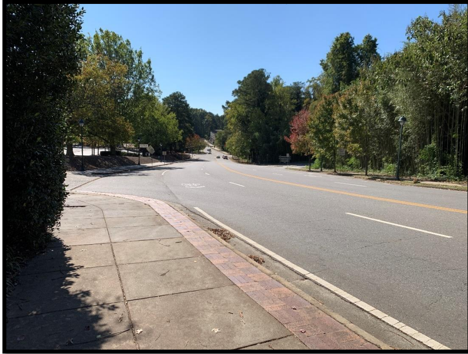
Photograph 11 – Sandy Springs Circle Facing South at Parkside Shops Accesses
