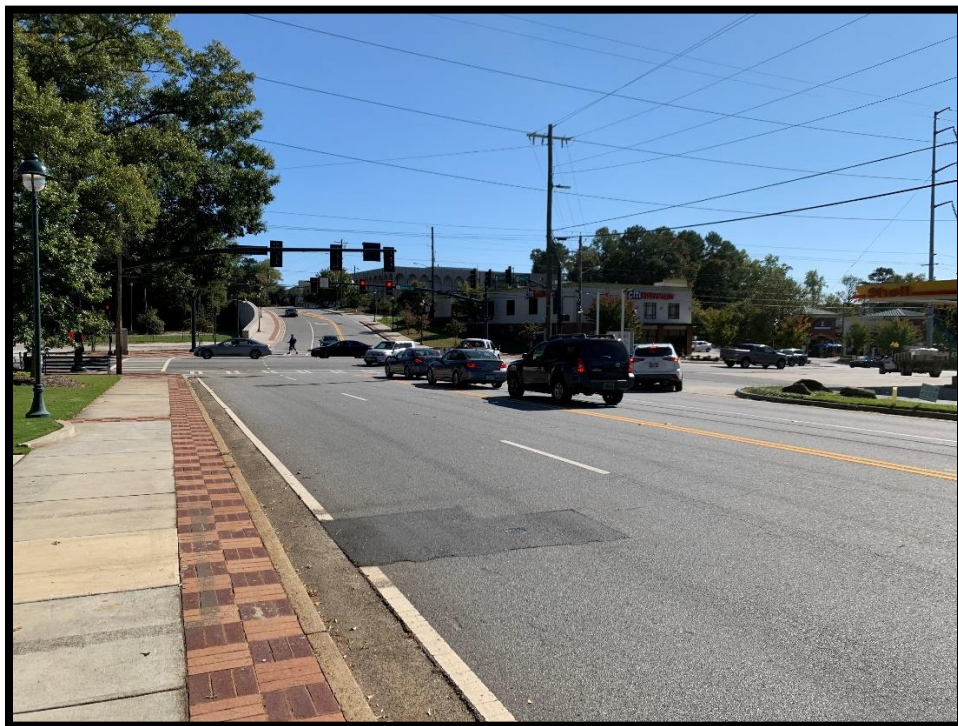
Photograph 6 – Cliftwood Drive Facing East at Roswell Road
