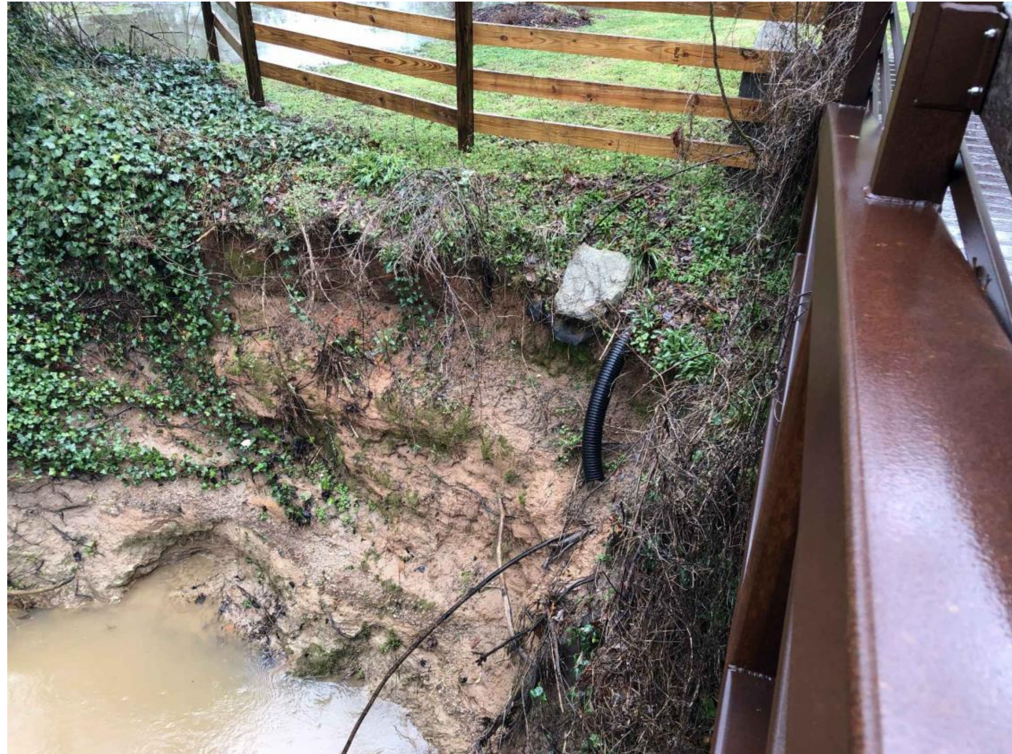
View west from bridge
