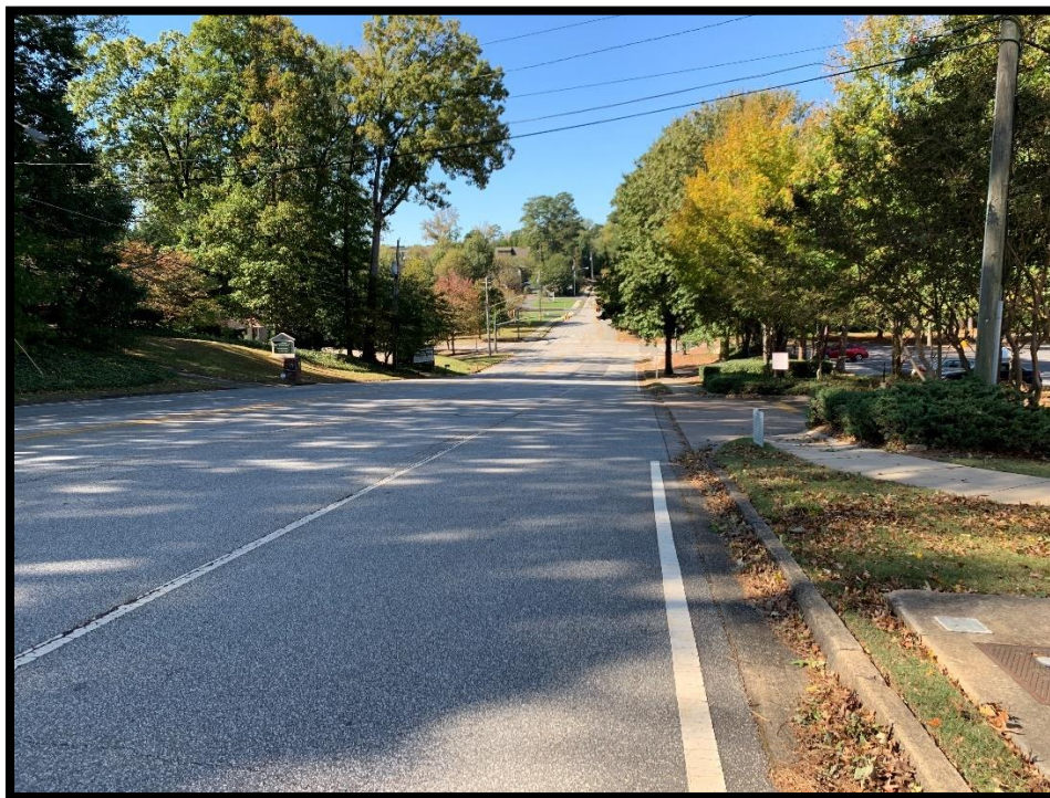
Photograph 8 – Cliftwood Drive Facing West at Parkside Shops West Access
