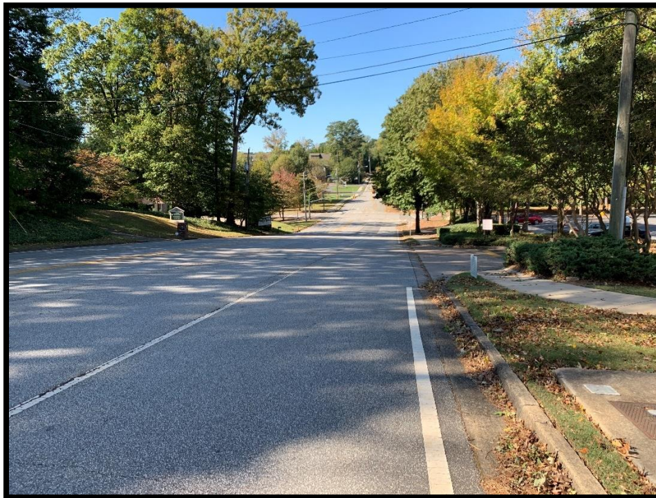
Photograph 8 – Cliftwood Drive Facing West at Parkside Shops West Access
