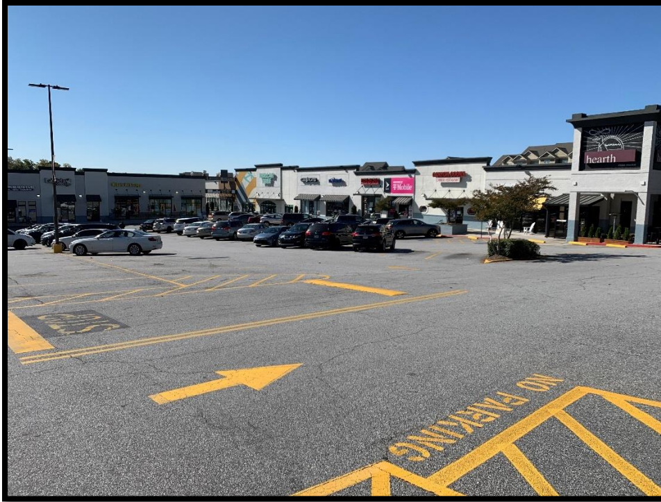
Photograph 13 – Hammond Exchange Parking Lot Incorrect Striping Colors
