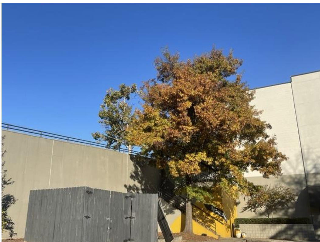
View of service area to the left of the theater entrance, facing northeast
