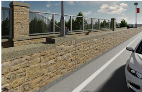
Interior Barrier Wall
