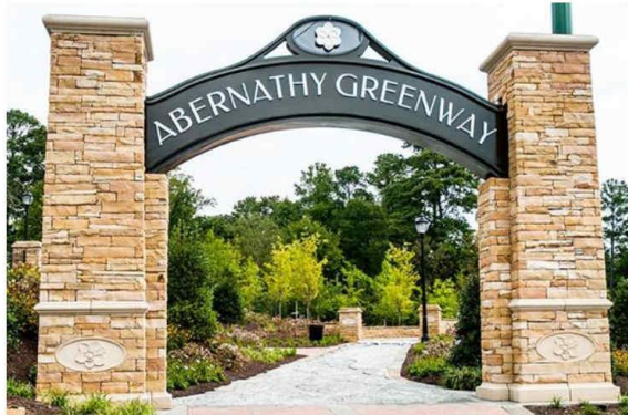
Abernathy Greenway Gateway Columns and Walls
