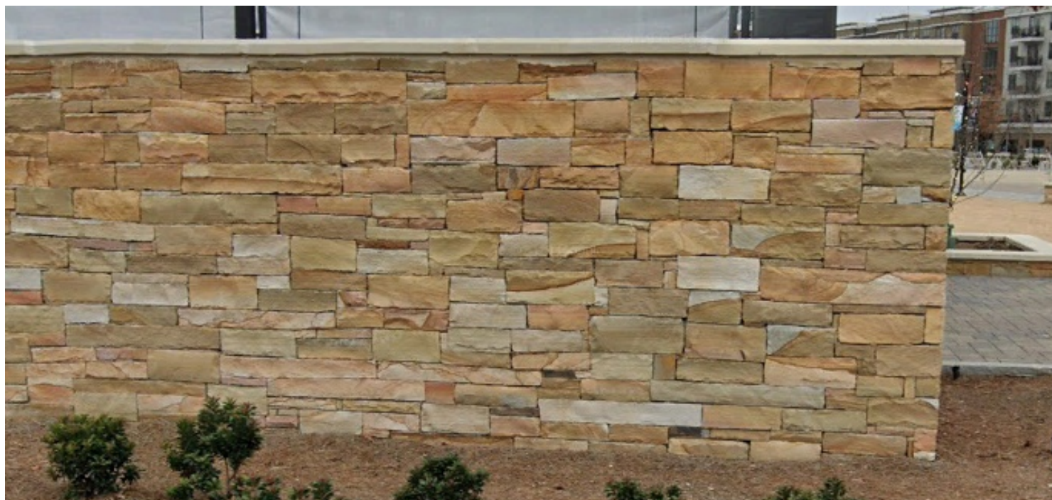
City of Sandy Springs City Hall Stacked Stone Walls
