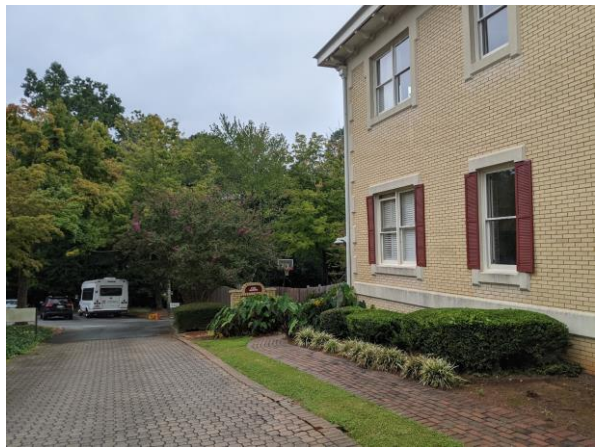
Side of building and rear of property from drive alley, facing west
