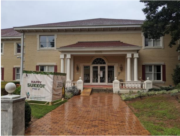
Side of building from drive alley, facing north
