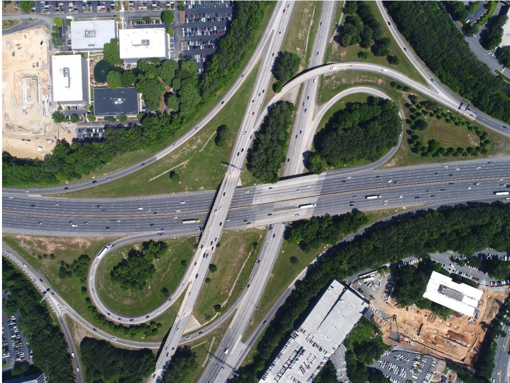
Interchange Before Construction
