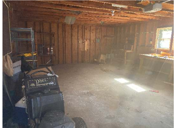
Interior of Detached garage
