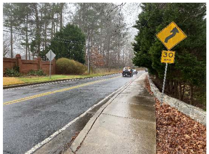
Looking southwest on Mount Vernon Rd.
