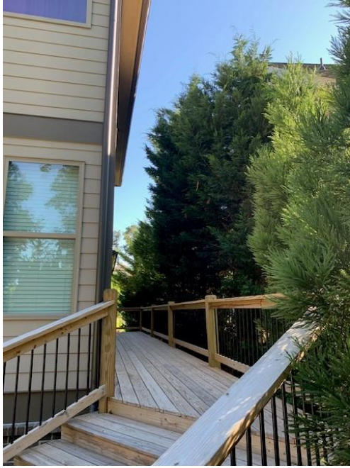
Current Extension (Level Across the Rear of the Home) with steps to the Pool Deck
