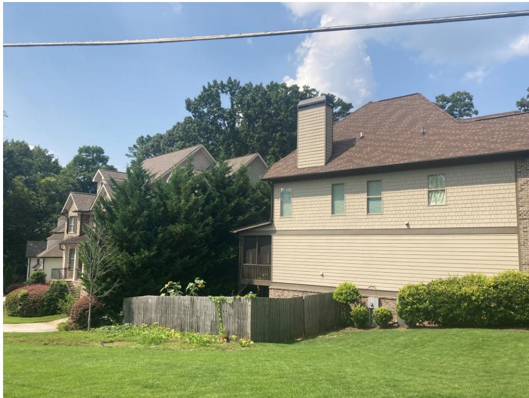
View northwest from Long Island Place (subject property to right)
