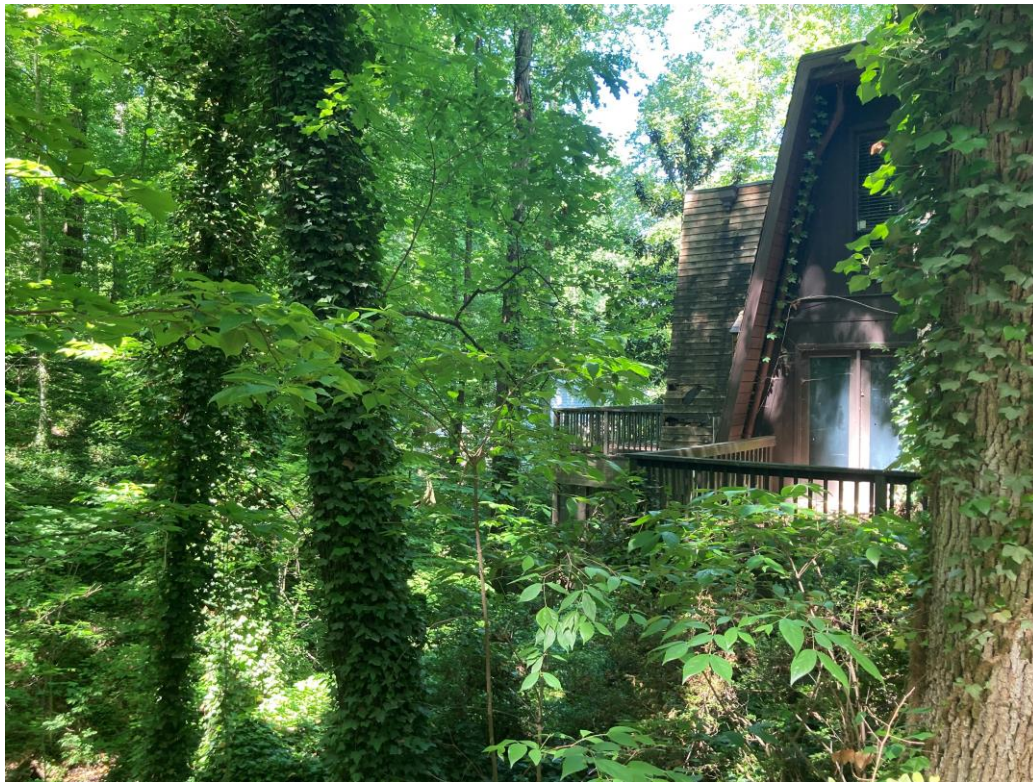
Decks on south side of residence
