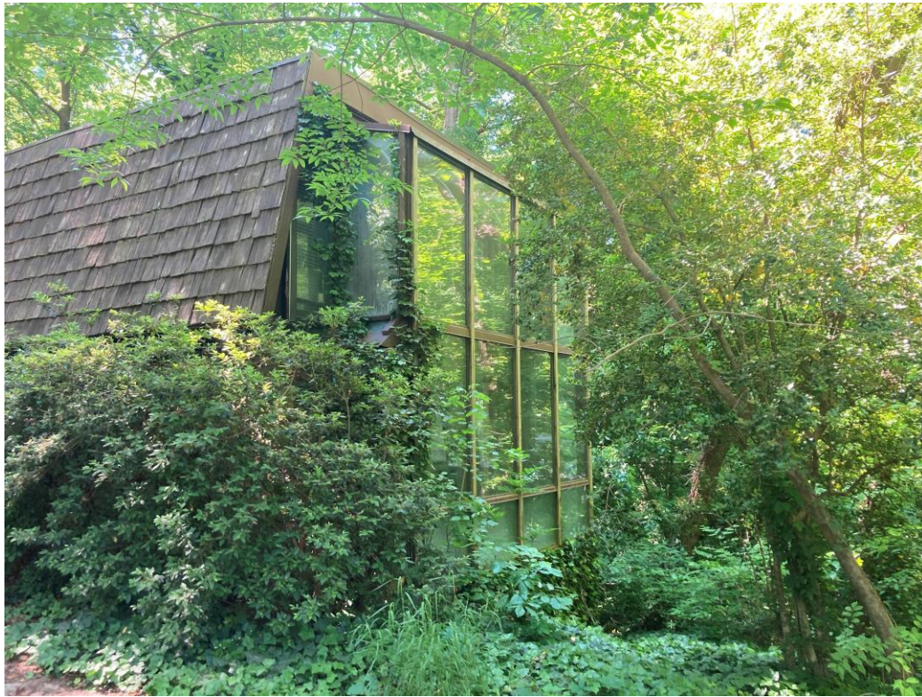
East side of residence
